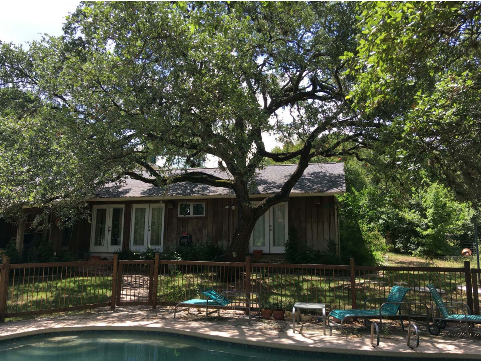
EXISTING HOME, NW CORNER
