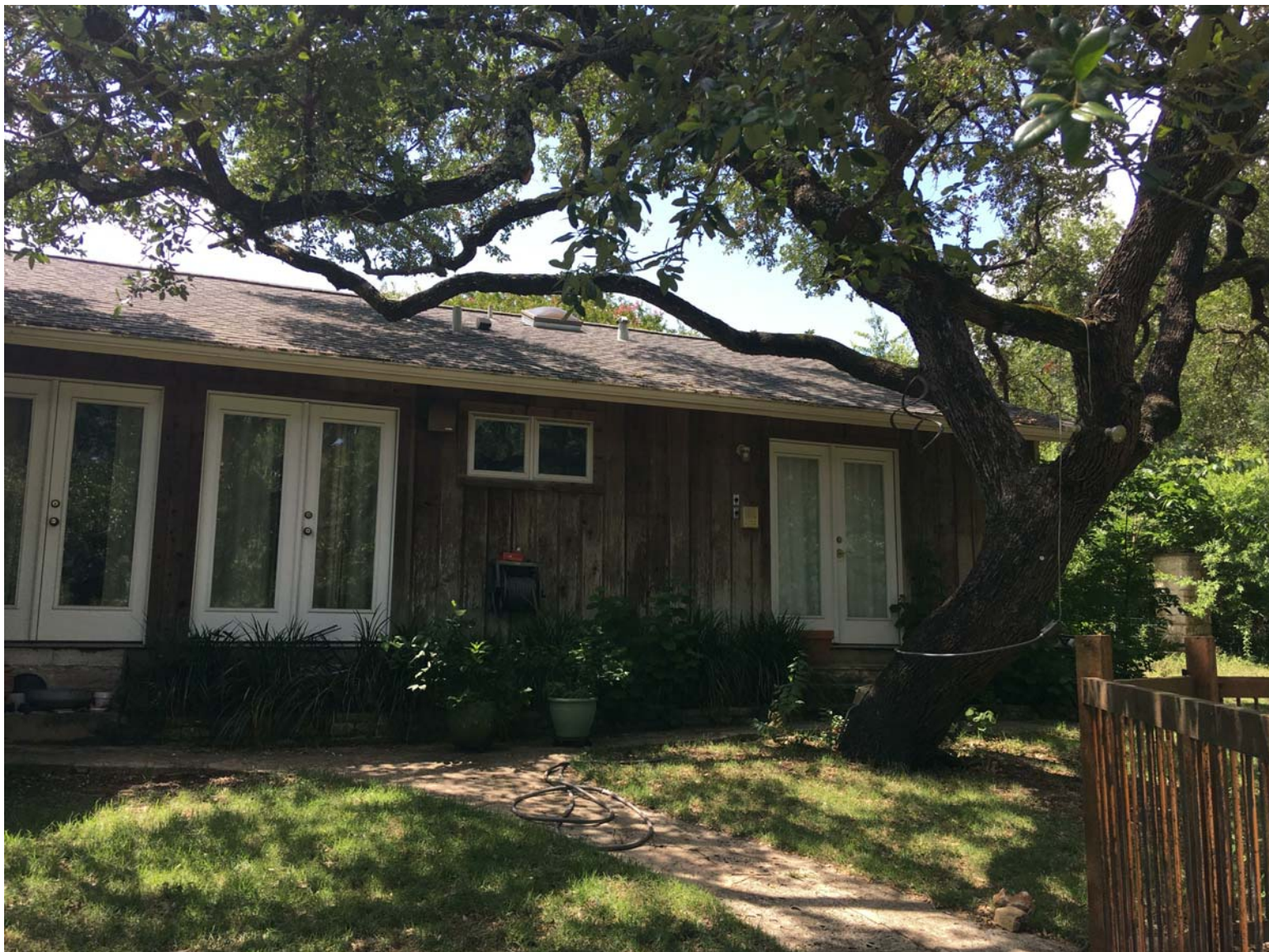
EXISTING HOME, NORTH ELEVATION
