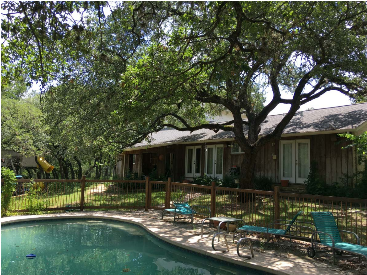
EXISTING HOME, NORTH ELEVATION
