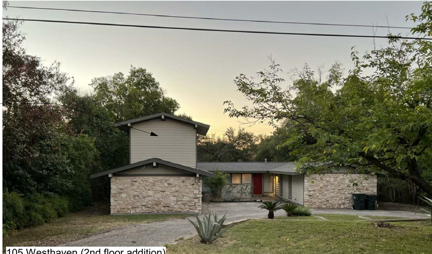
105 Westhaven (2nd floor addition)
