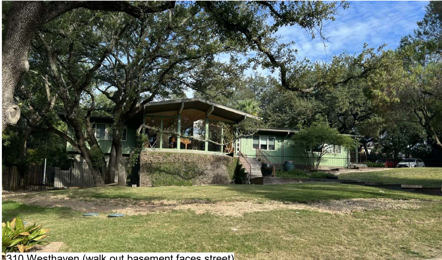
310 Westhaven (walk out basement faces street)
