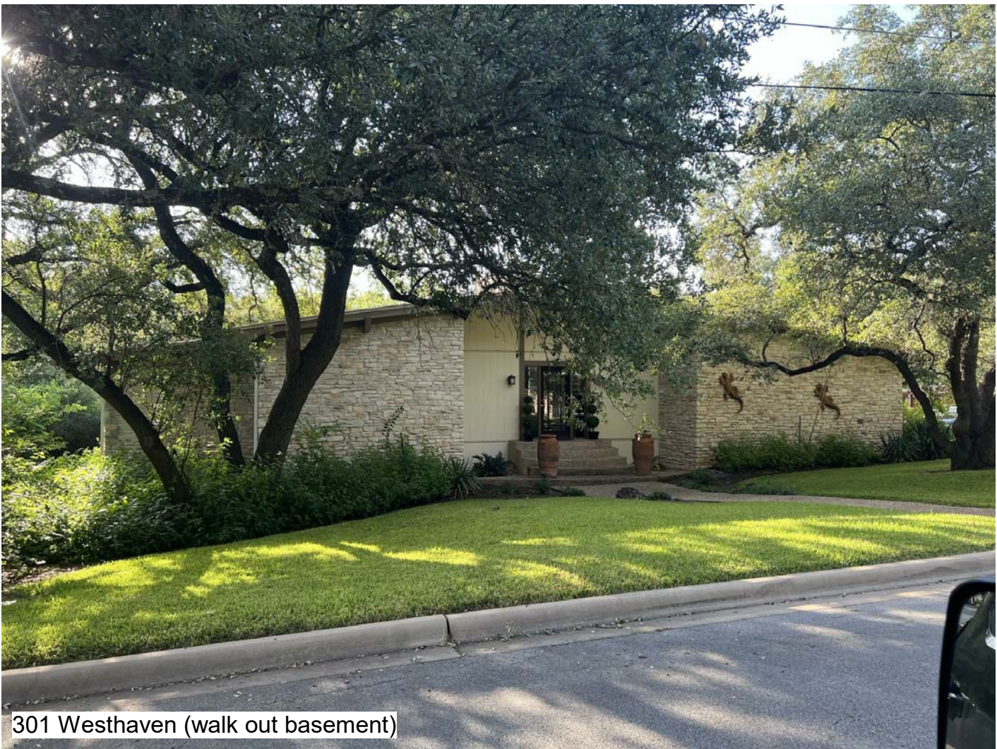
301 Westhaven (walk out basement)
