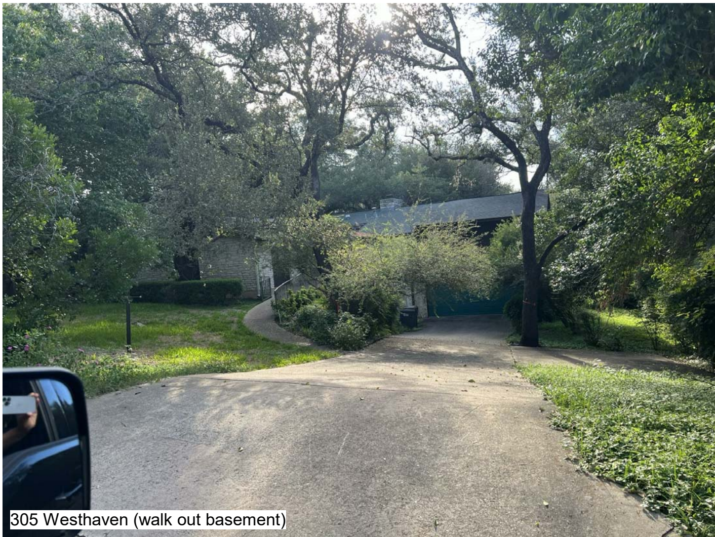
305 Westhaven (walk out basement)
