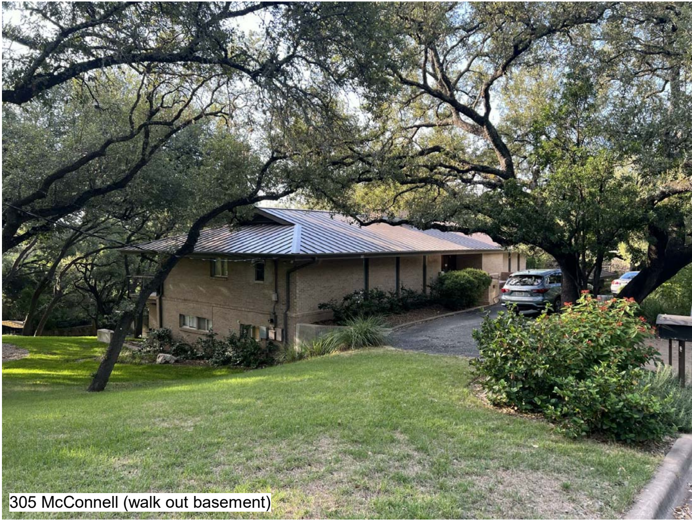
305 McConnell (walk out basement)
