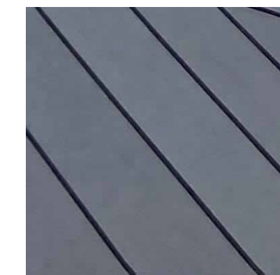
STANDING SEAM METAL ROOF TO MATCH EXISTING
