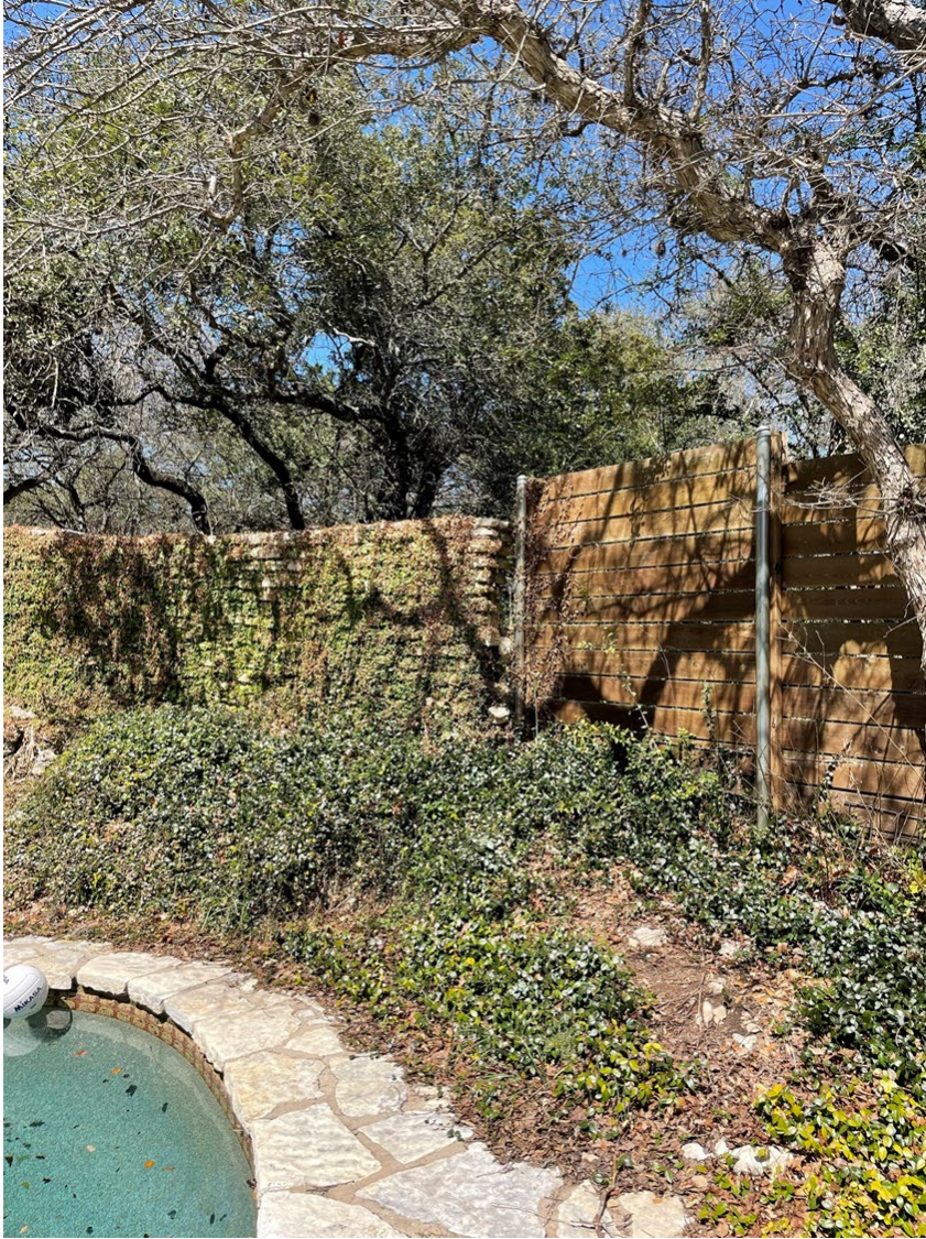
VIEW 9 – WOOD FENCE TO BE REMOVED THIS AREA, STONE WALL TO REMAIN
