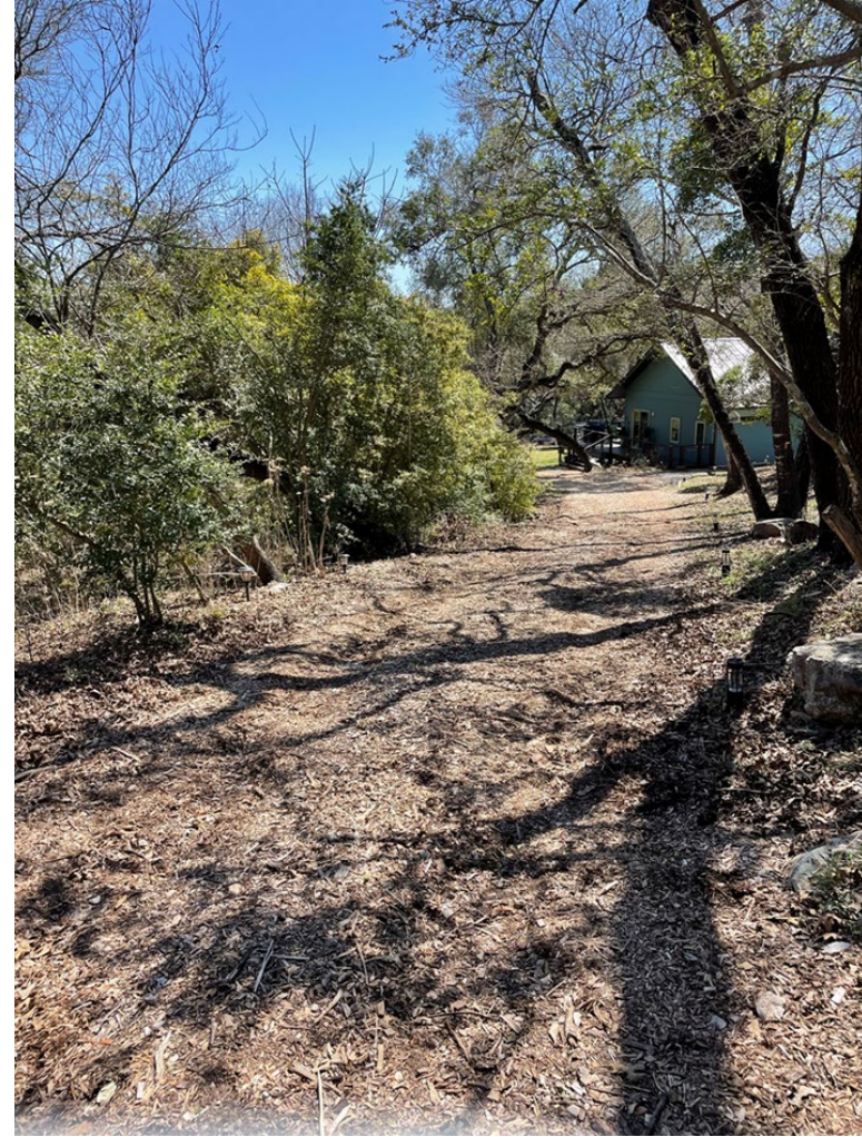
VIEW 14 – HIGHLY ERODED MULCH DRIVE TO LOWER ADU PROPOSED TO BE IMPROVED WITH PERVIOUS CONCRETE
