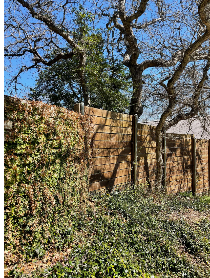
VIEW 10 – WOOD FENCE TO BE REMOVED THIS AREA, STONE WALL TO REMAIN, 6" DIA. OAK TO BE REMOVED AND REPLACED
