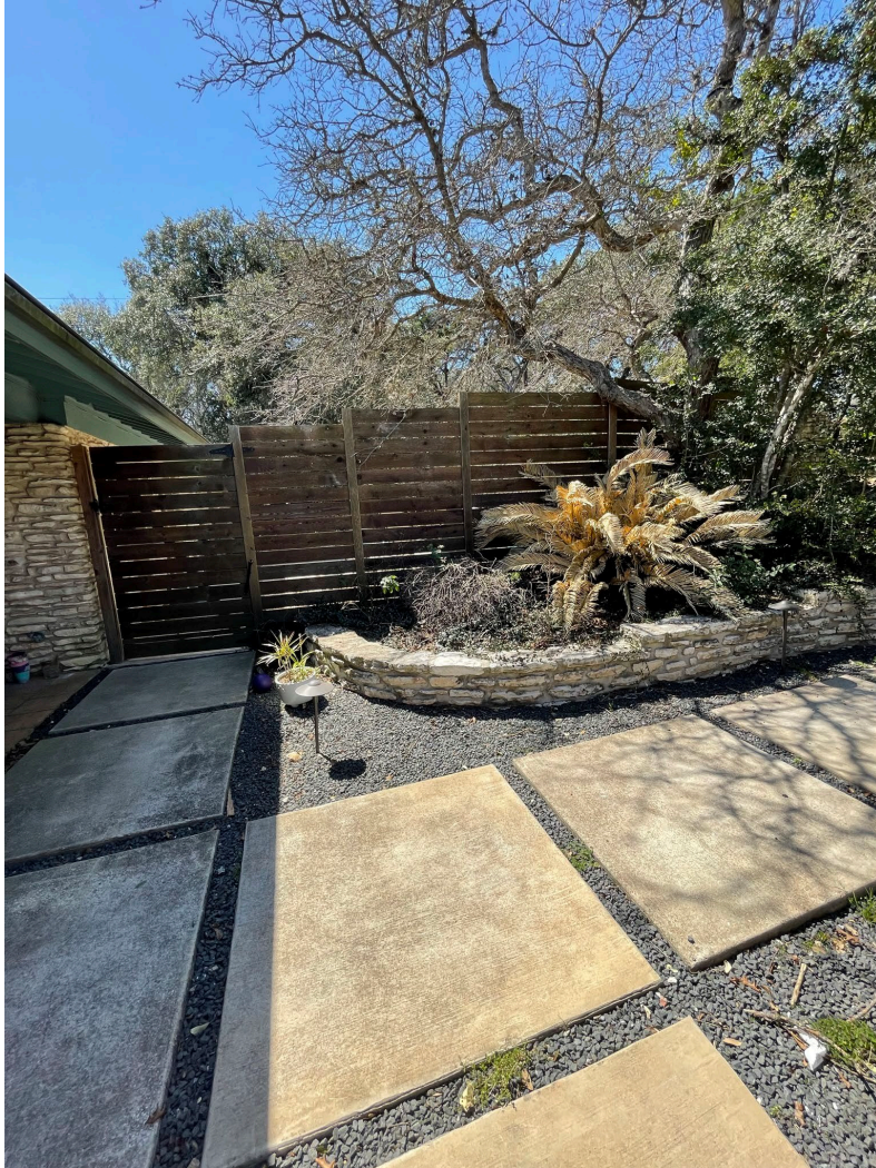
VIEW 5 – WOOD GATE AND FENCE TO BE REMOVED THIS AREA, STONE WALL TO REMAIN, LARGE TREE TO BE PROTECTED
