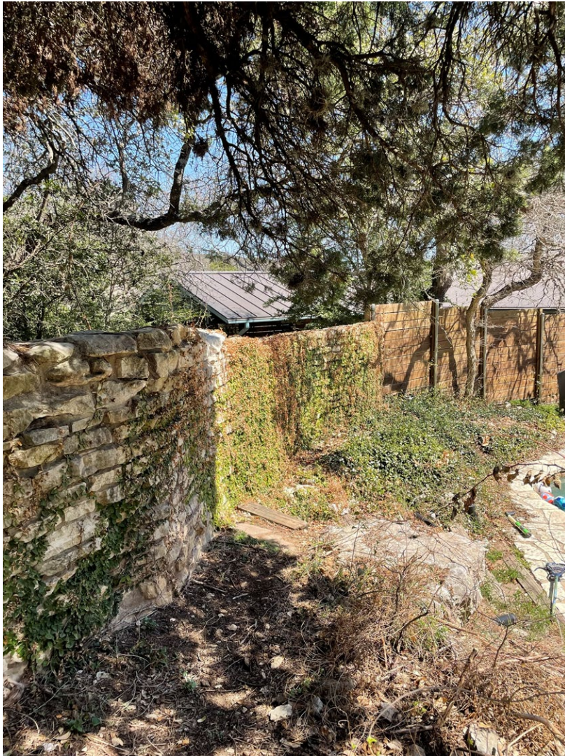
VIEW 11 – STONE WALL TO REMAIN, WOOD FENCE TO BE REMOVED THIS AREA
