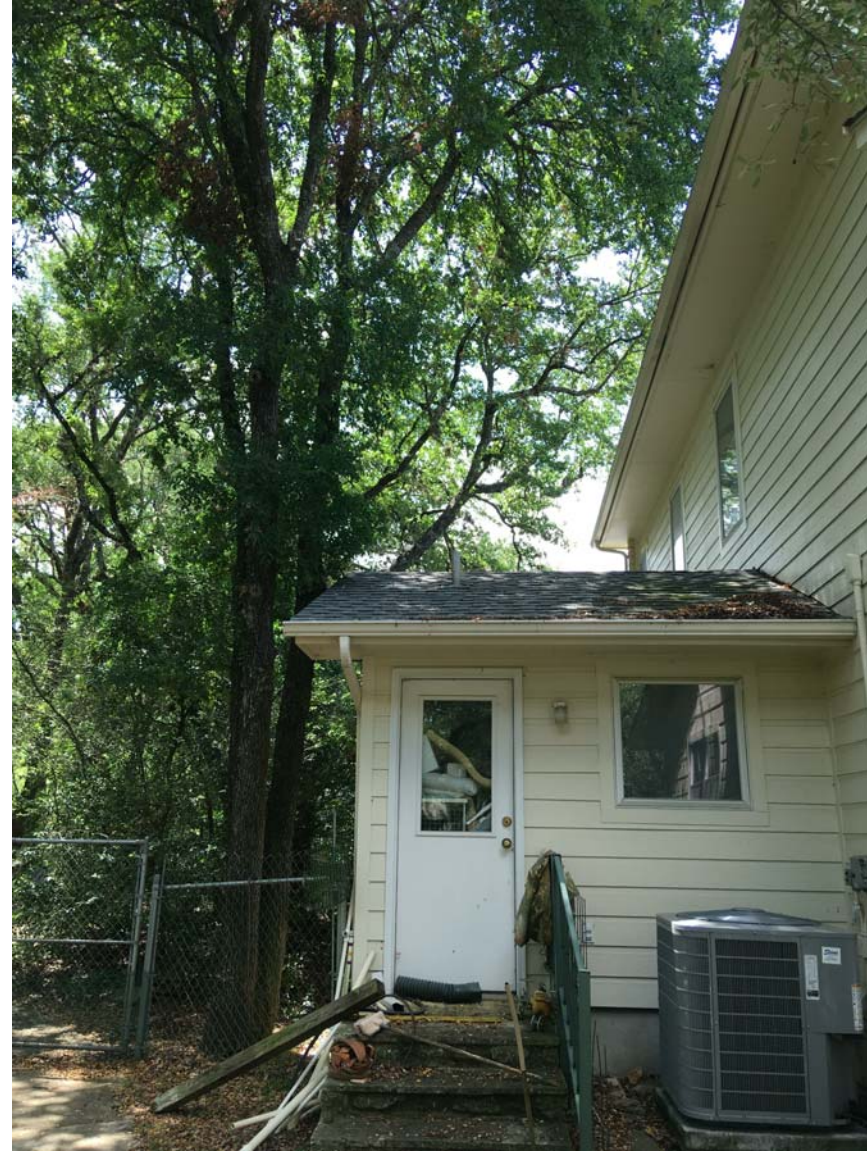
EXISTING HOME, NE CORNER
