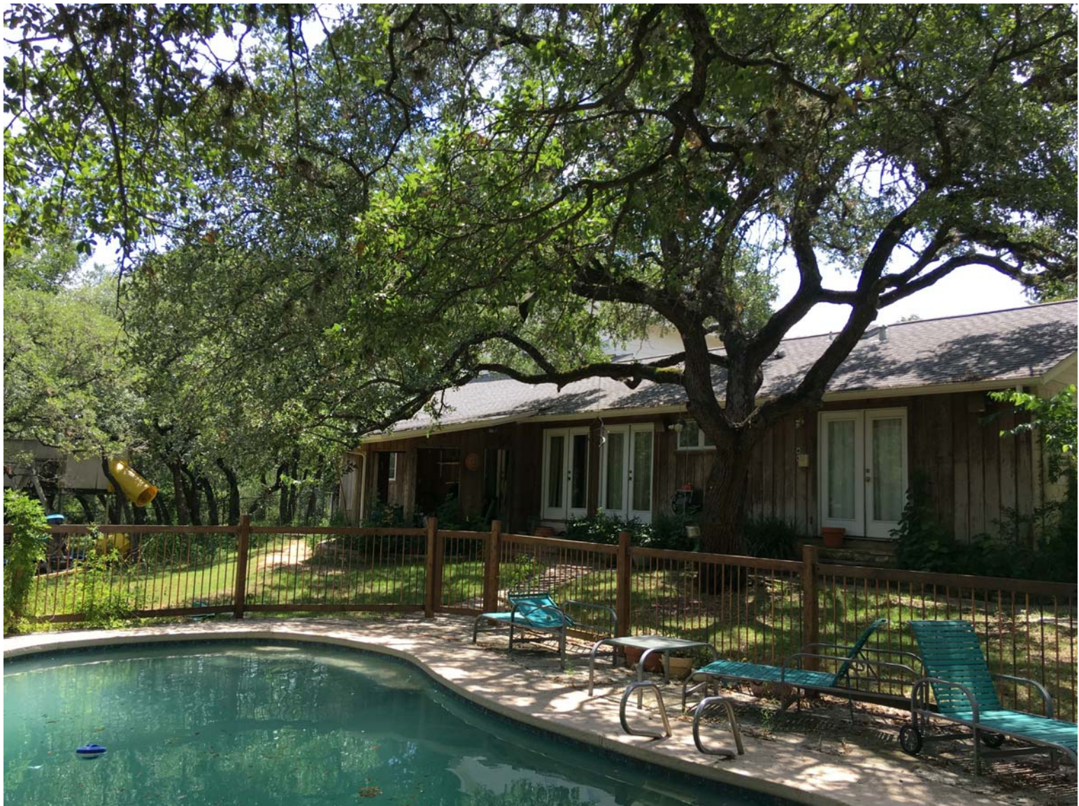
EXISTING HOME, NORTH ELEVATION
