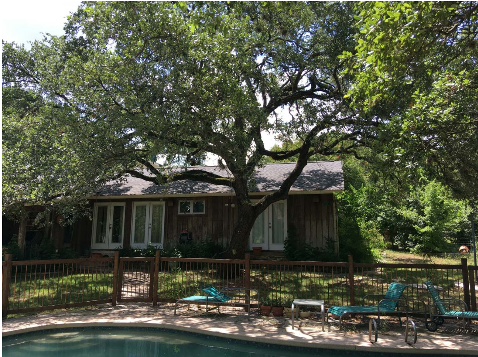
EXISTING HOME, NW CORNER
