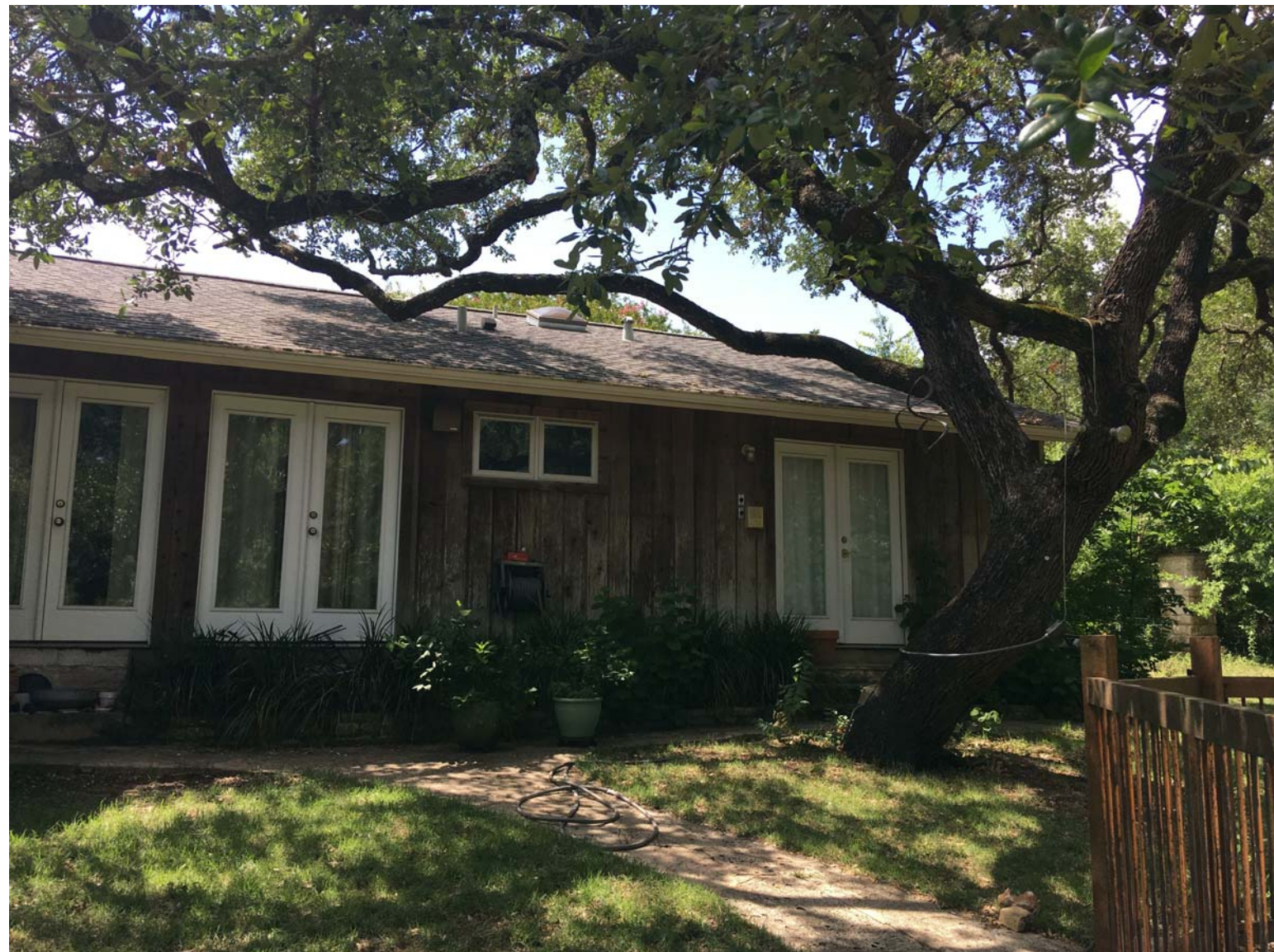
EXISTING HOME, NORTH ELEVATION
