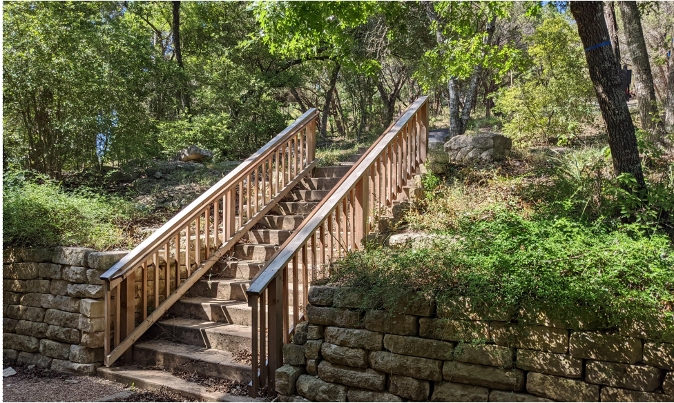
EXISTING PHOTO B
