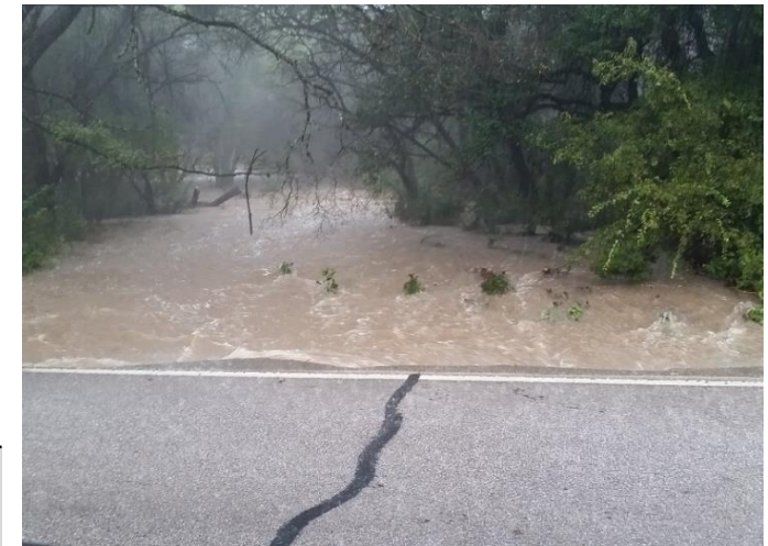
October 30, 2015 flood event, Little Bee Creek at Westlake Drive
