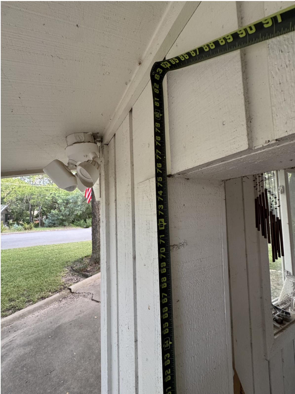
Photo 1: Interior - existing sloped roof structure at exterior wall (tape measure shown)
