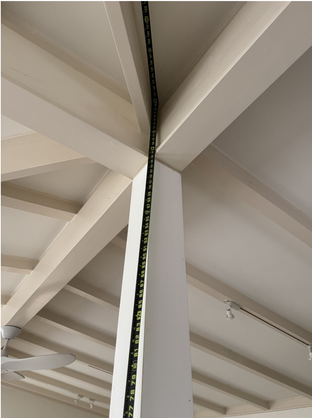
Photo 4: Interior - vaulted ceiling peak at clerestory windows (tape measure shown)
