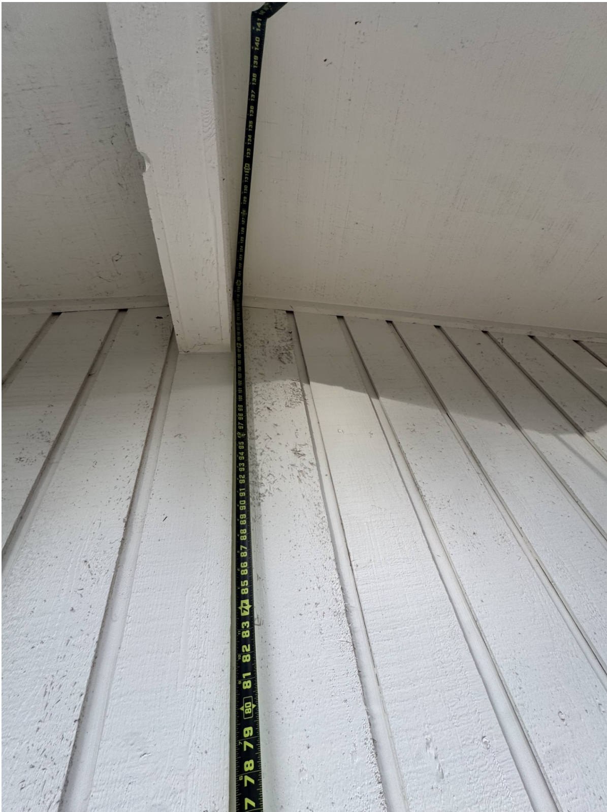
Photo 9: Exterior - carport / entry header clearance (tape measure shown)
