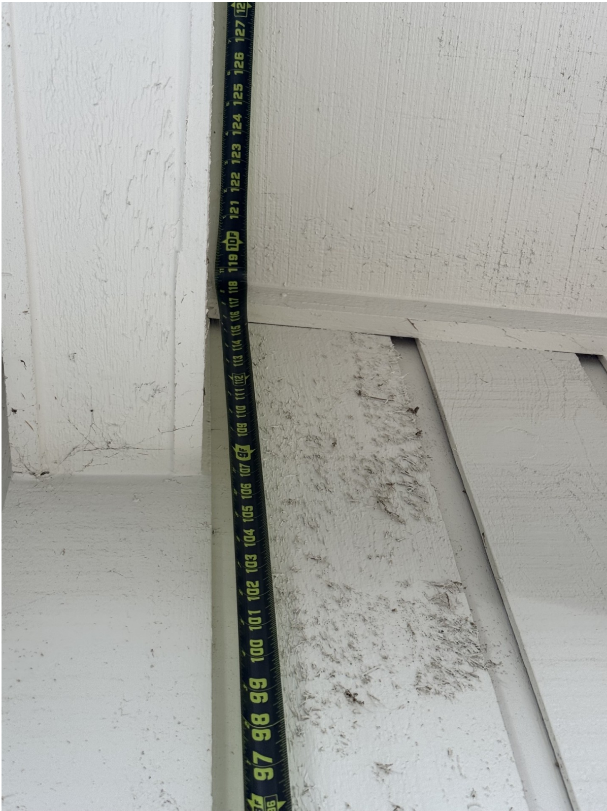
Photo 8: Exterior - existing eave / roof edge height at exterior wall (tape measure shown)
