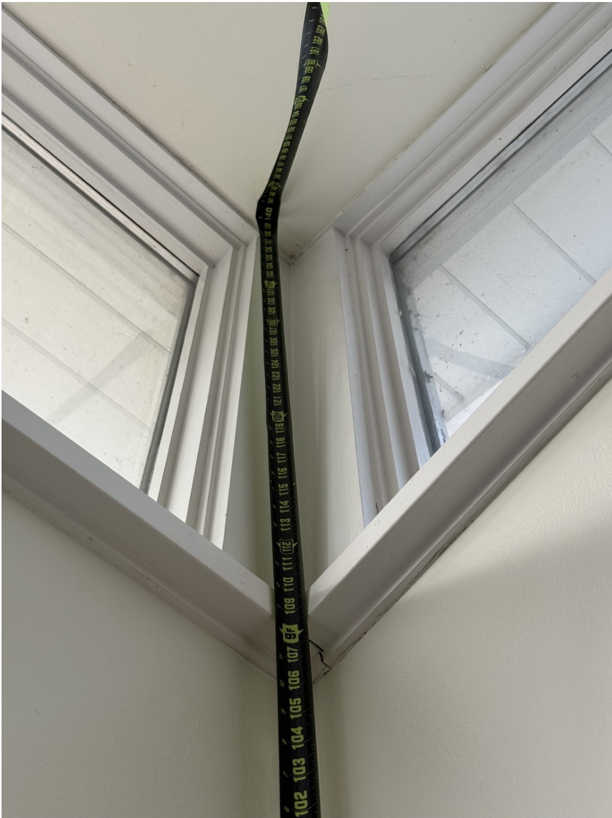
Photo 5: Interior - vaulted ceiling peak between clerestory windows (tape measure shown)
