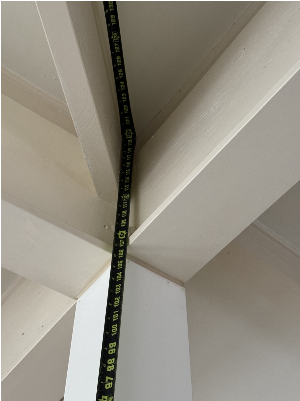
Photo 3: Interior - existing ceiling height at wall (tape measure shown)
