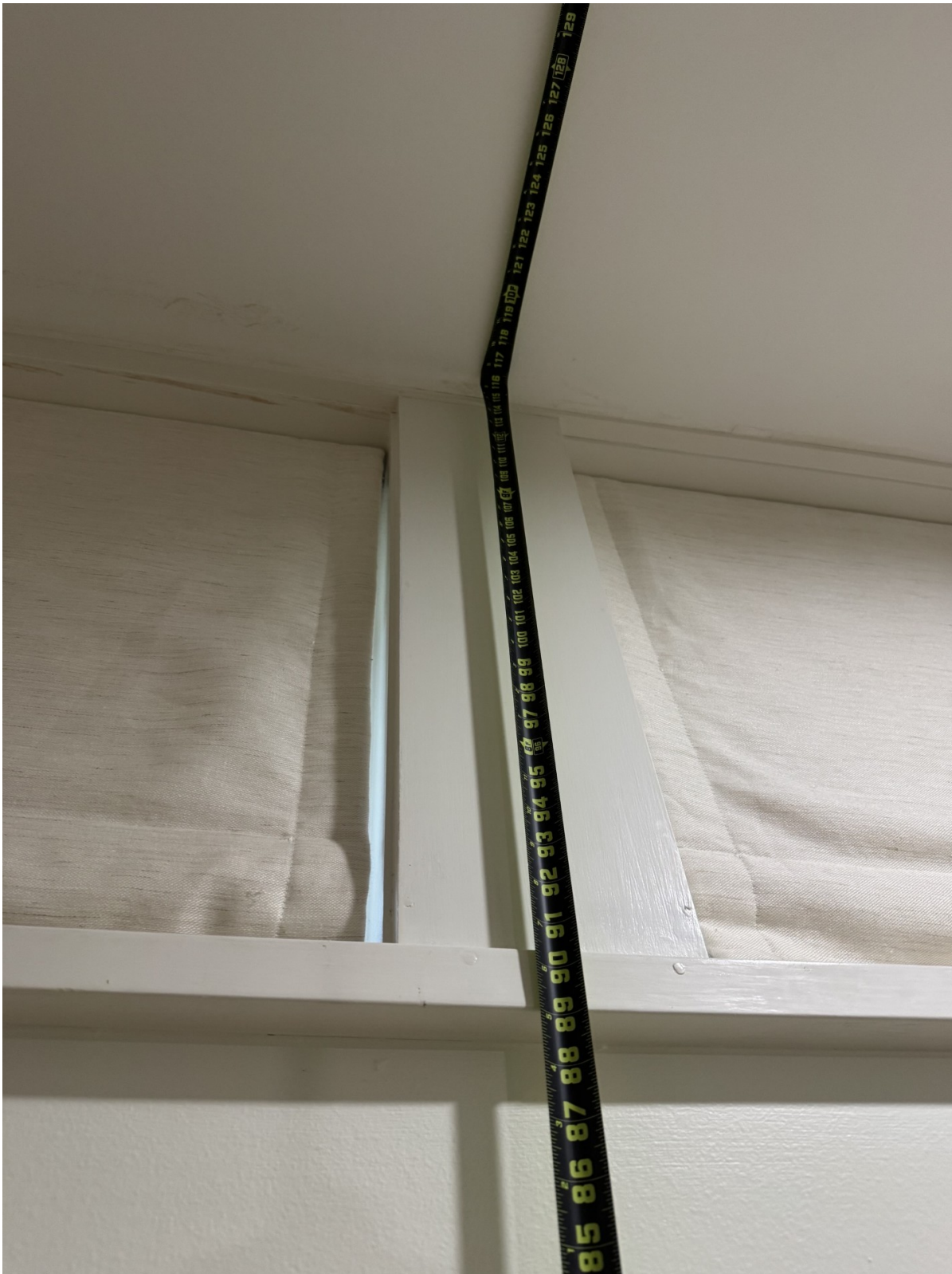
Photo 7: Interior - exposed beam ceiling at ridge beam (tape measure shown)
