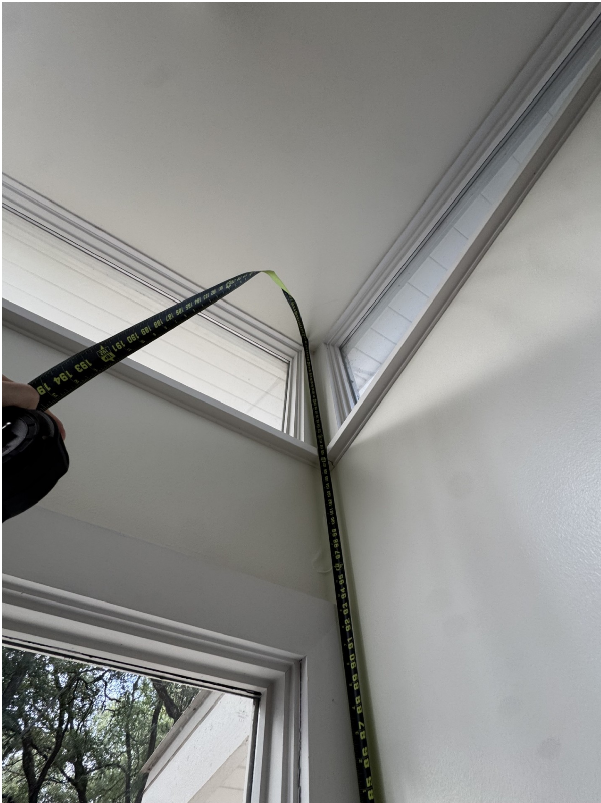
Photo 6: Interior - exposed beam ceiling at ridge (tape measure shown)
