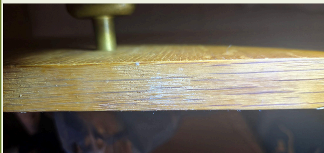
Suspected mold on top edge of master vanity drawer.
