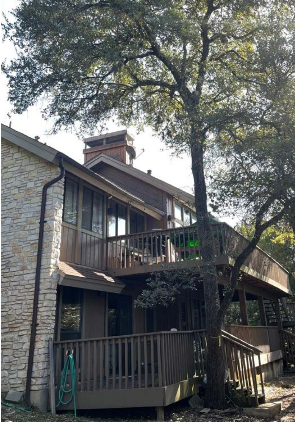
# 5051 Live Oak (Multiple branches) - 16.75" Removal due to proximity to dwelling.
