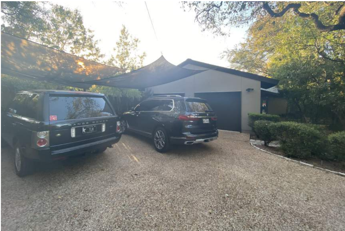
EXIST. CONDS.-EAST-GARAGE NTS 2
