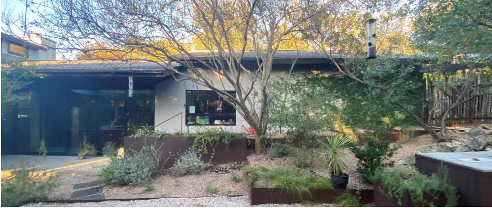
EXIST. CONDS.-SOUTH-EXISTING HOUSE NTS 9
