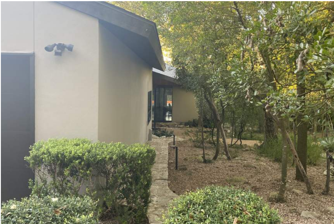
EXIST. CONDS.-EAST- WALKWAY NTS 3
