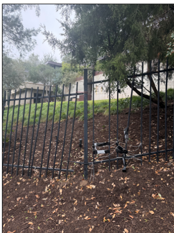
Existing/old 54" fence being replaced
