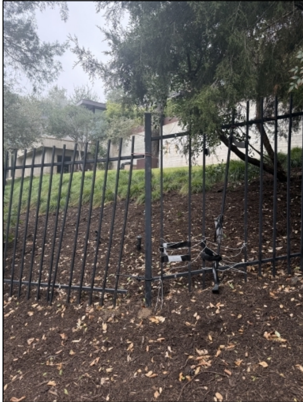
Existing/old 54” fence being replaced
