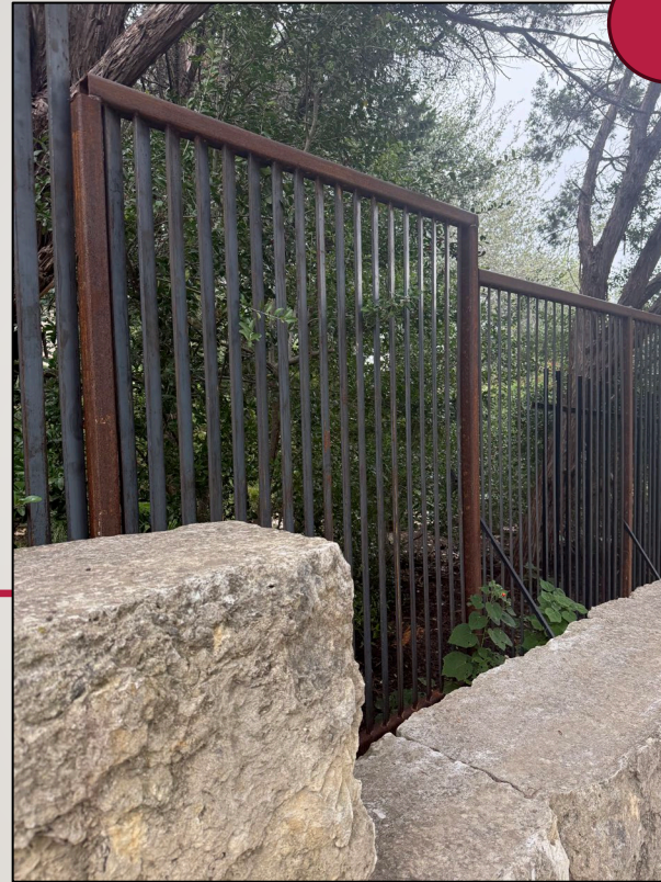
New fence sections installed before shutdown
