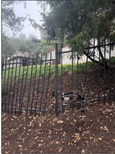
Existing/old 54” fence being replaced
