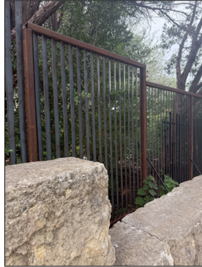
New 54” fence sections installed before shutdown
