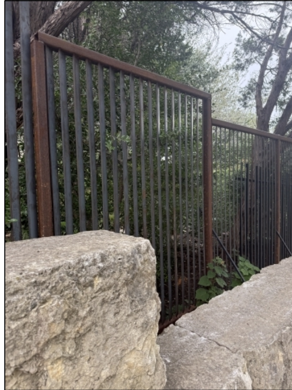
New 54” fence sections installed before shutdown
