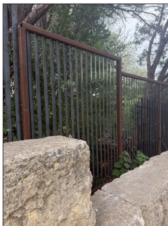
New 54" fence sections installed before shutdown
