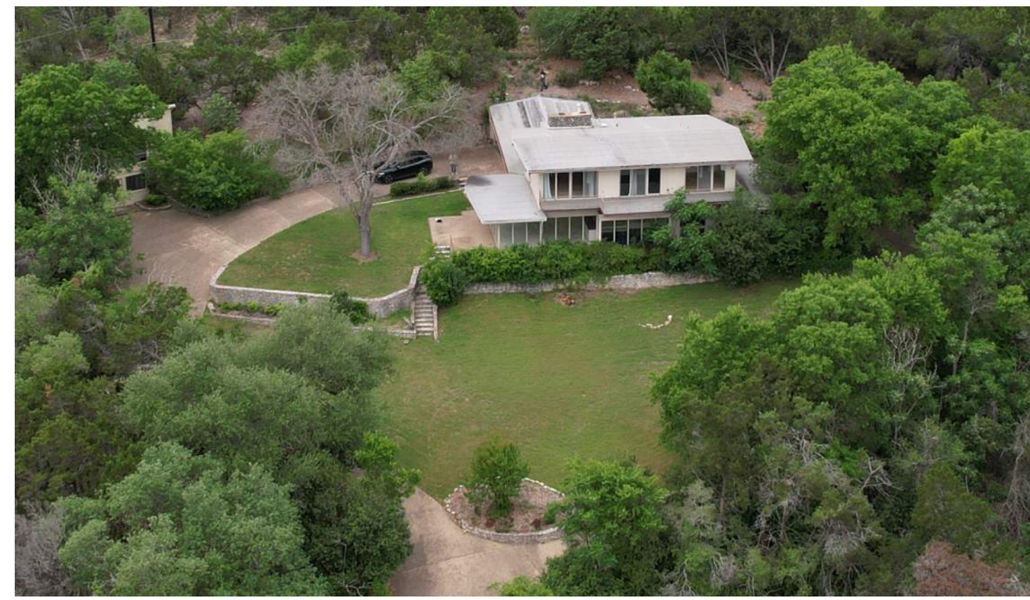
IMAGE OF EXISTING TWO STORY HOUSE AND CARPORT
