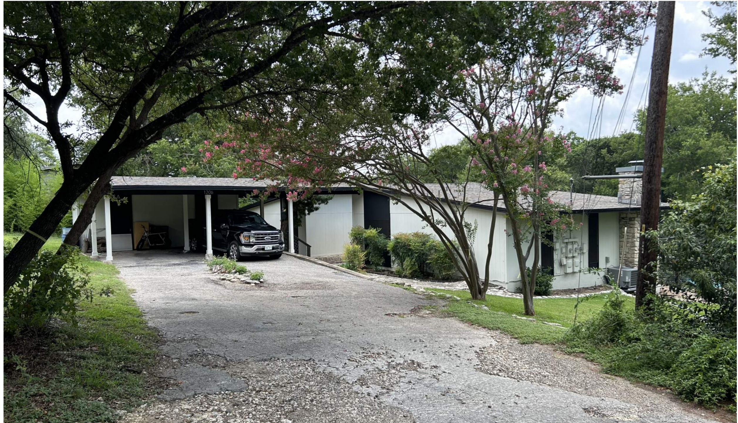
Existing Building Exterior
