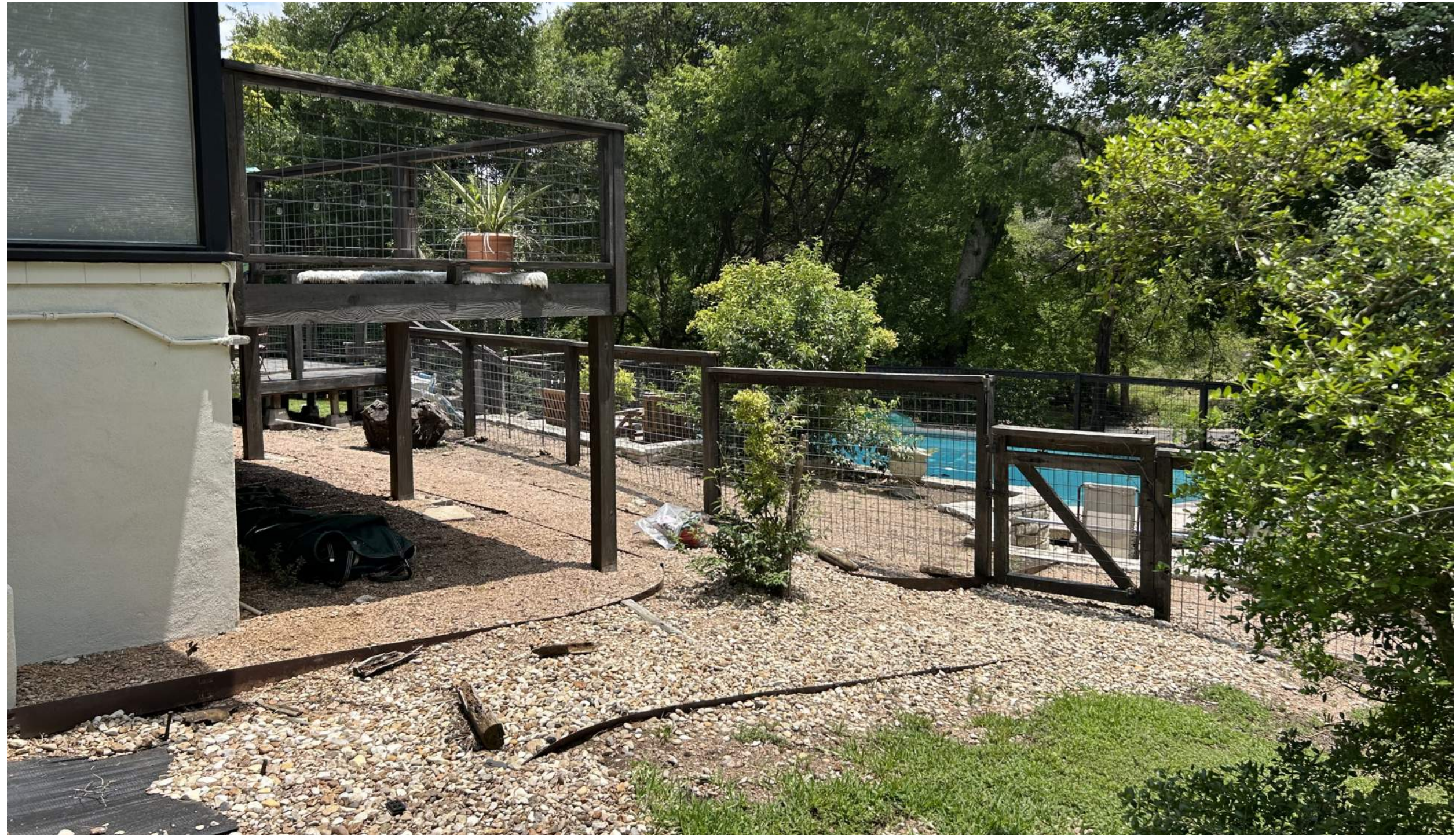
Existing Building Exterior
