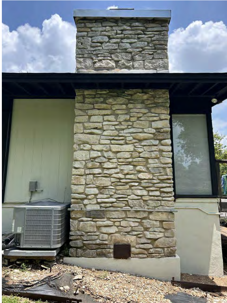
Existing Building Exterior
