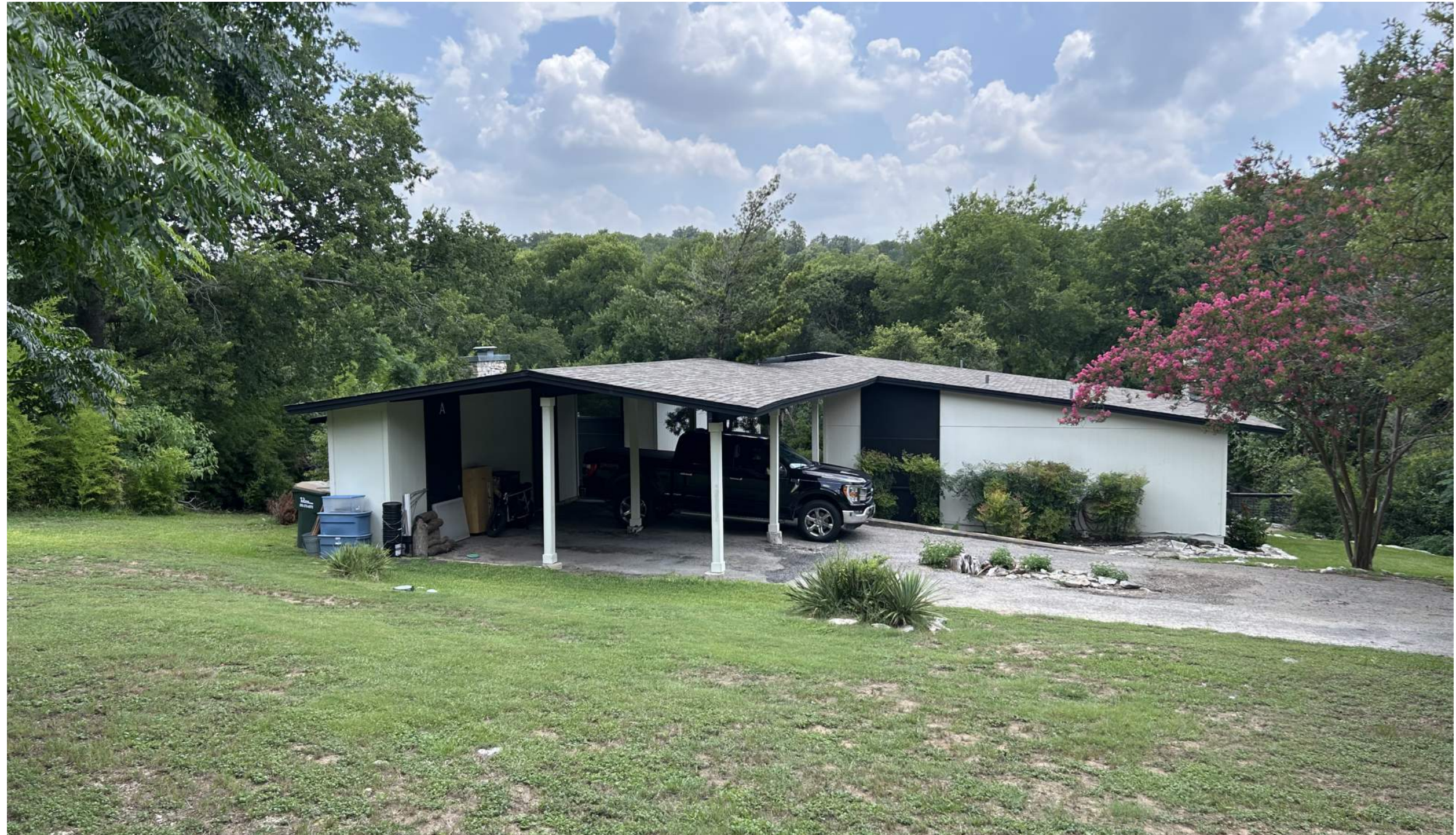
Existing Building Exterior
