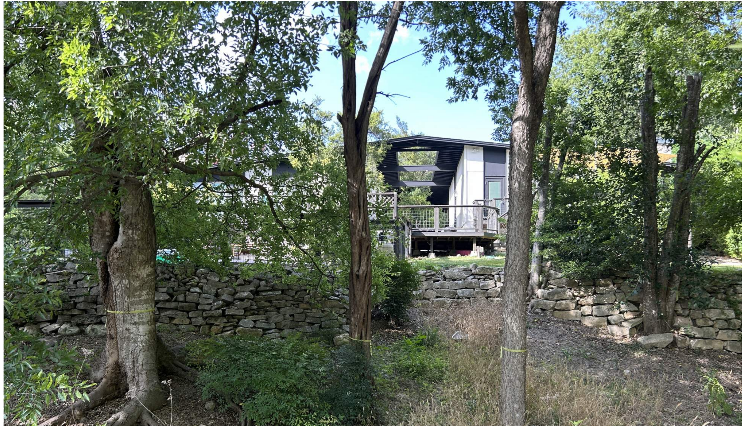
Existing Building Exterior
