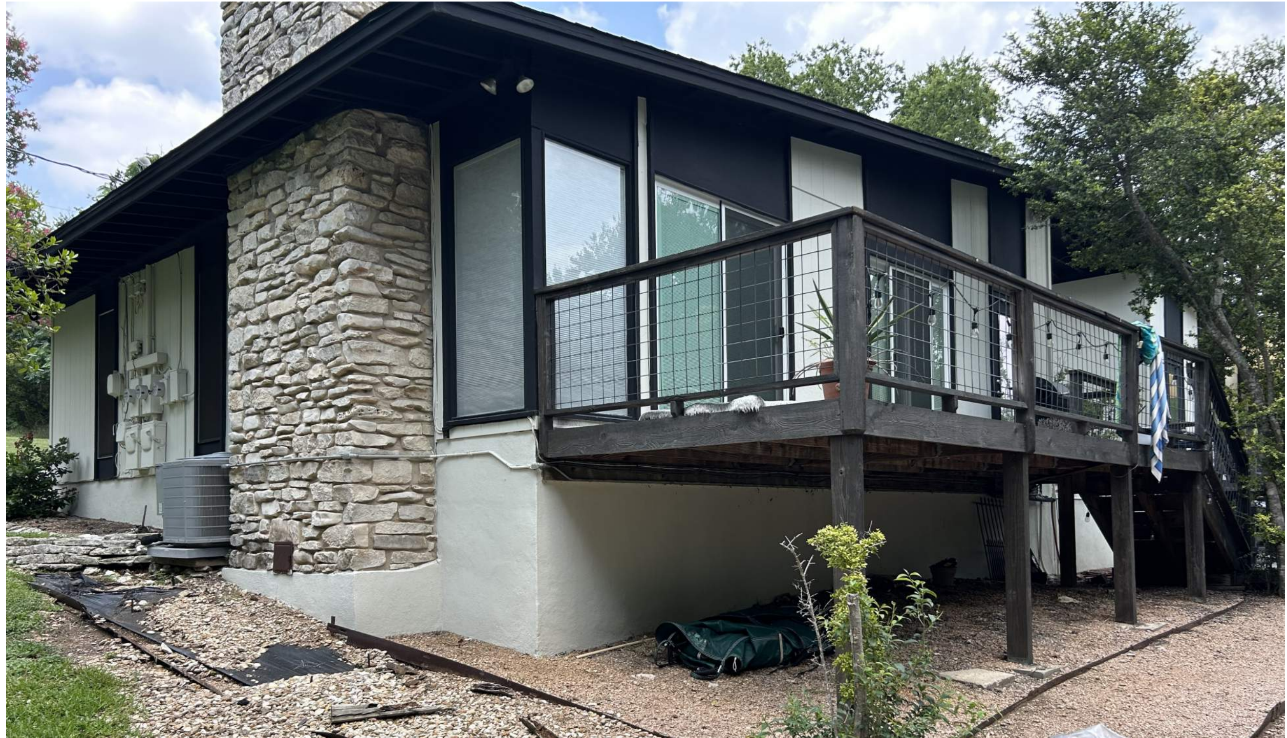
Existing Building Exterior
