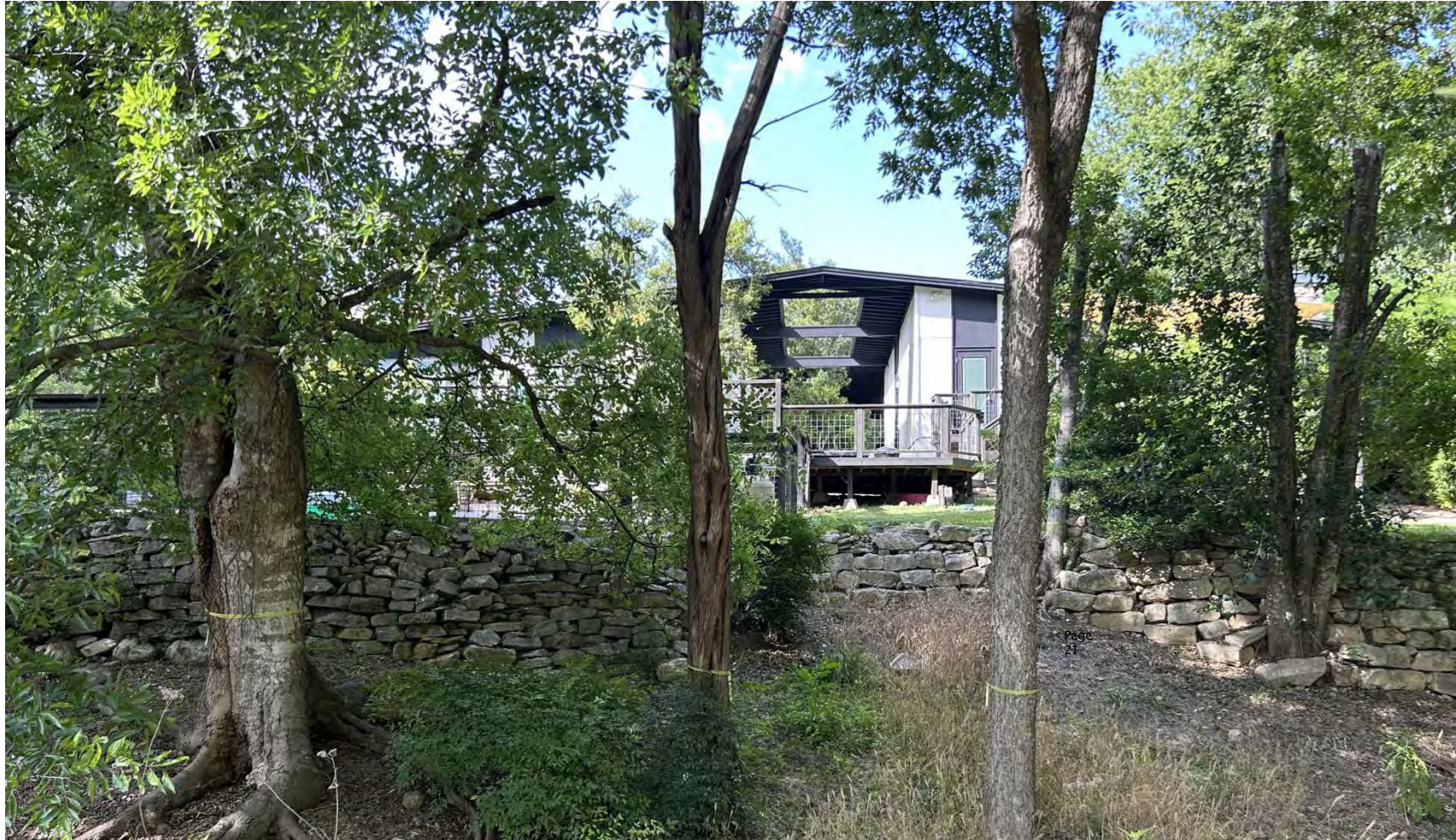
Existing Building Exterior
