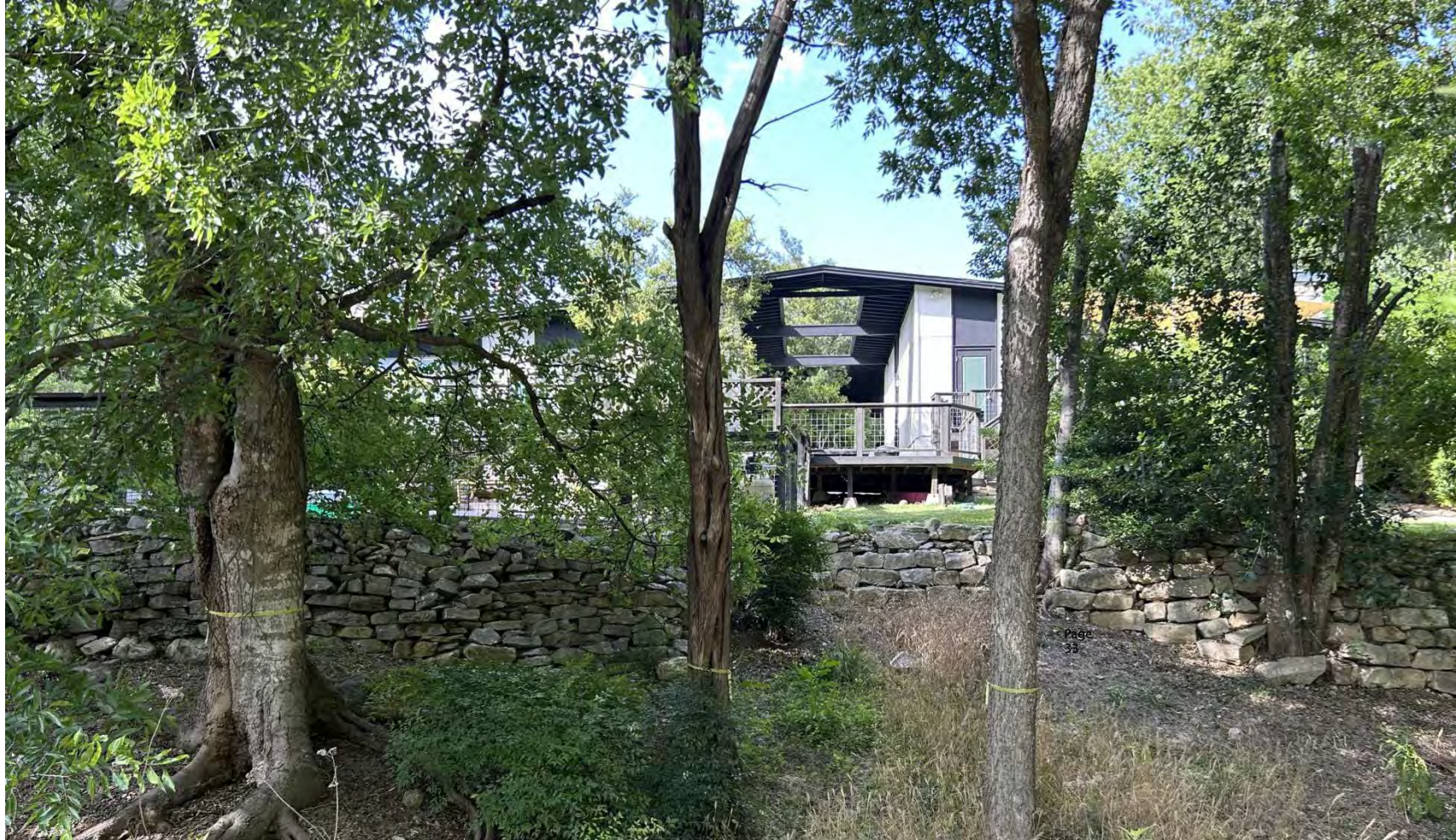
Existing Building Exterior
