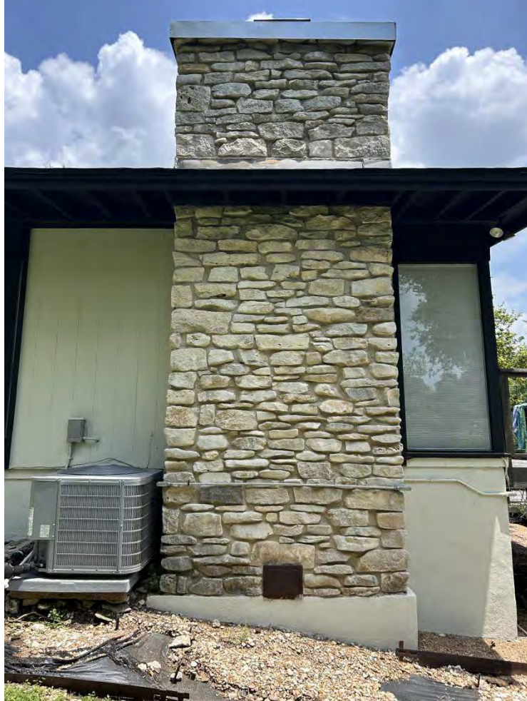
Existing Building Exterior
