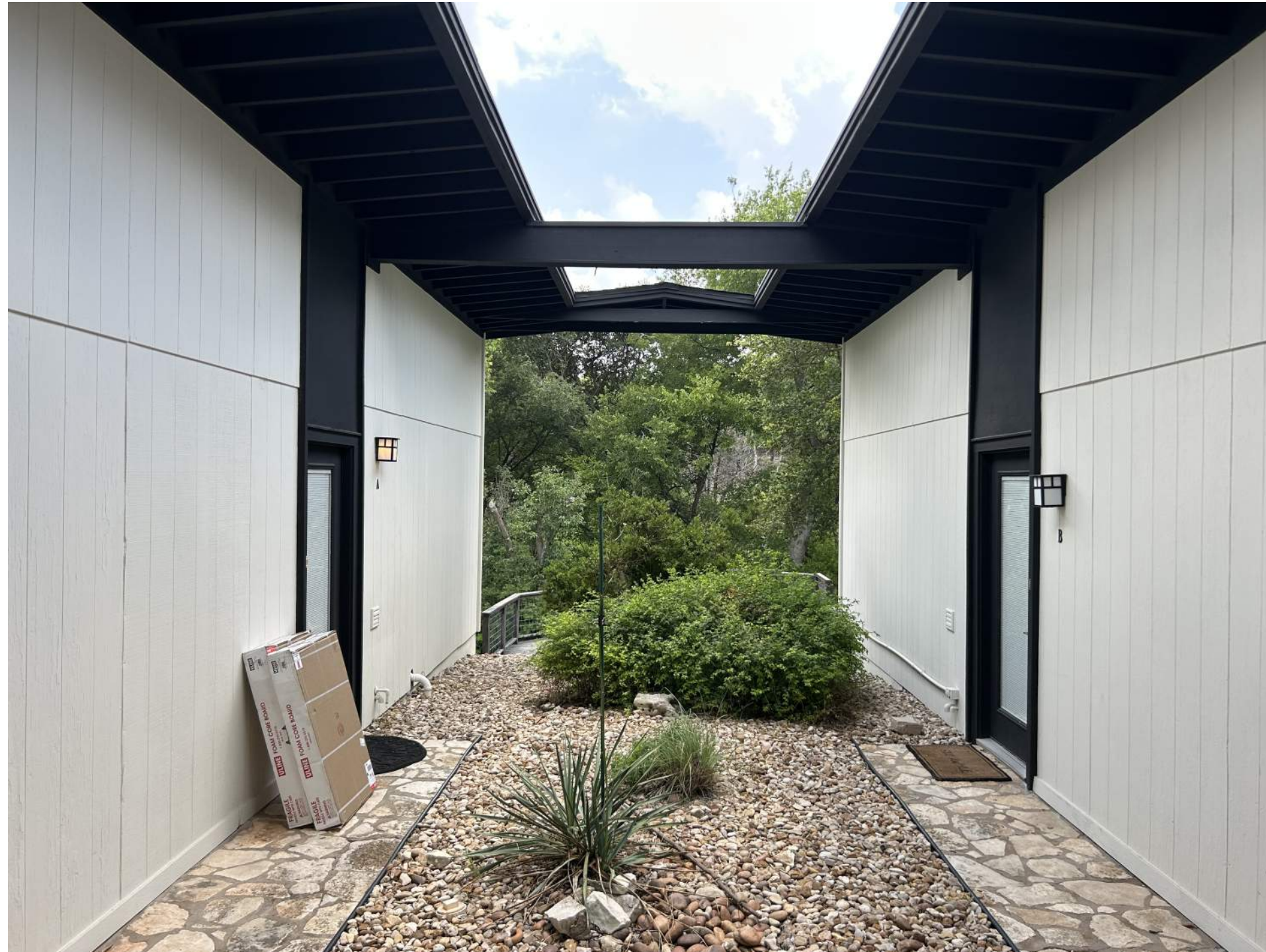
Existing Building Exterior
