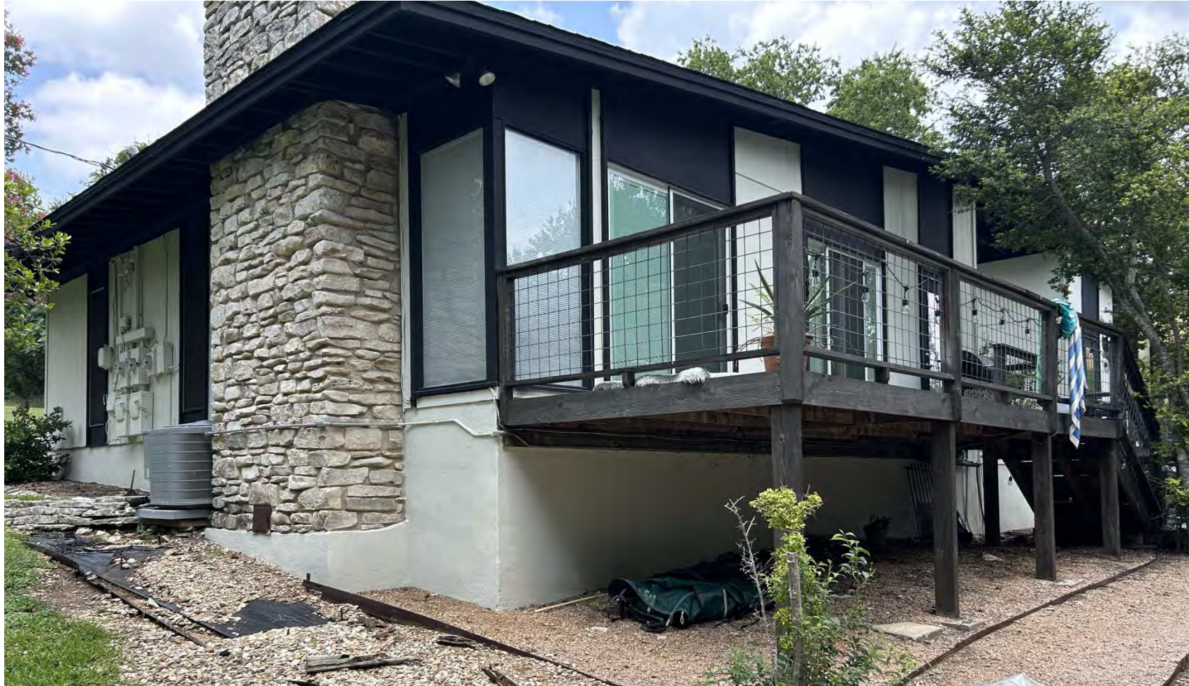
Existing Building Exterior
