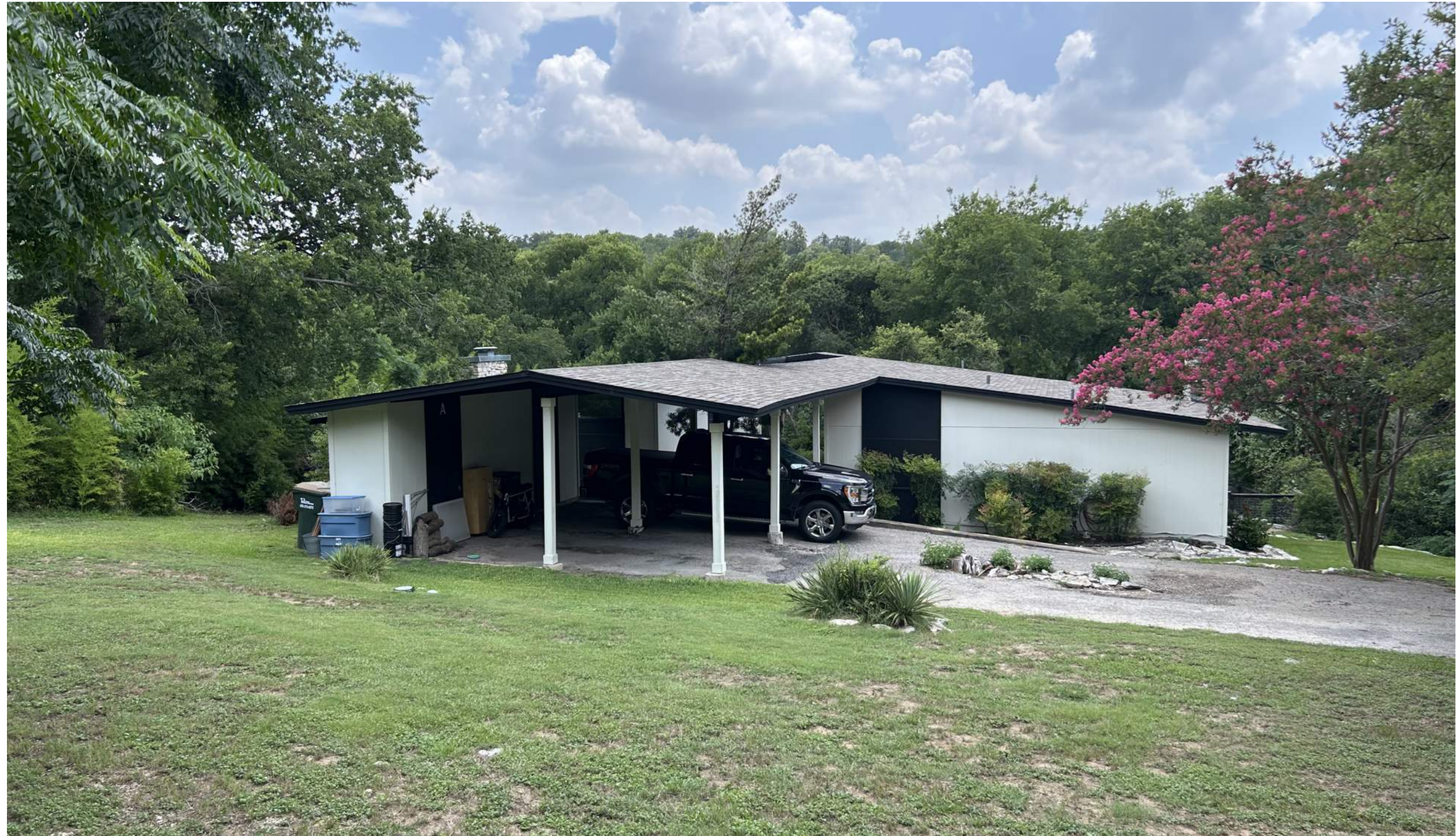
Existing Building Exterior
