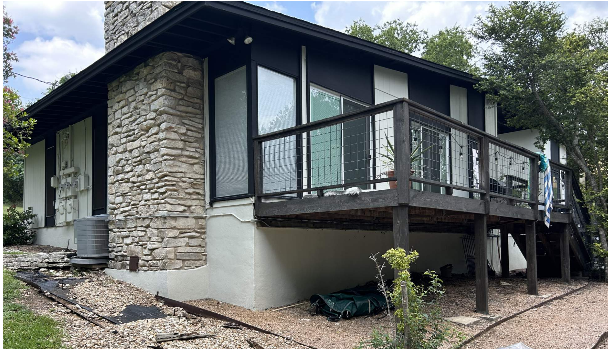
Existing Building Exterior
