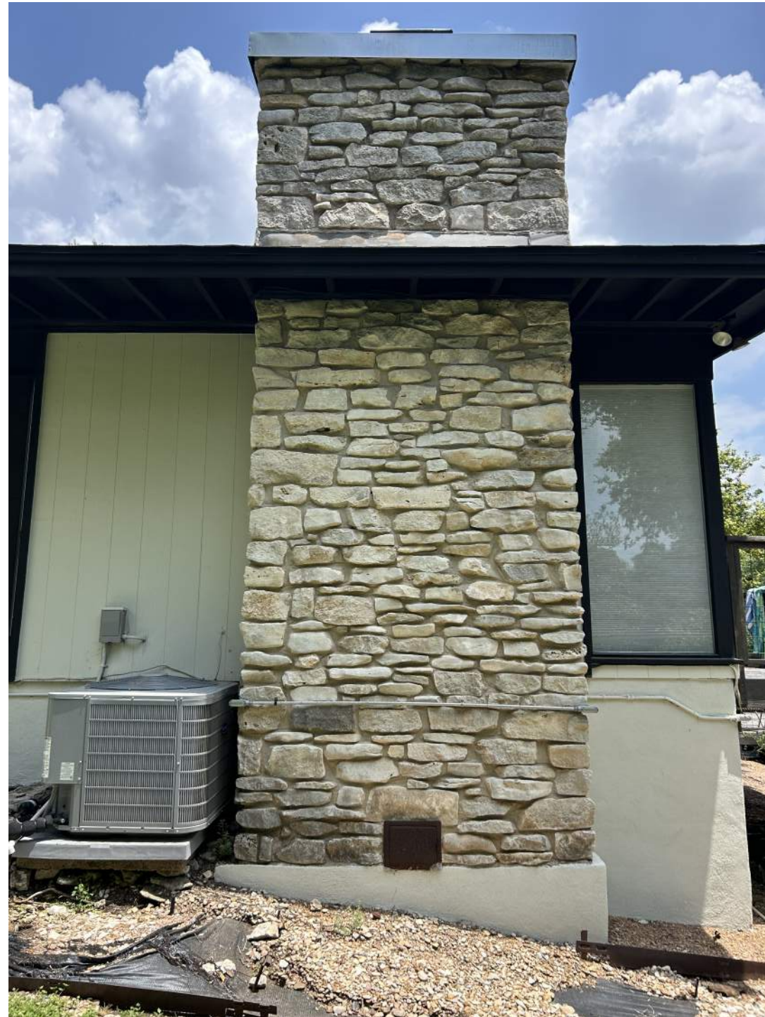
Existing Building Exterior
