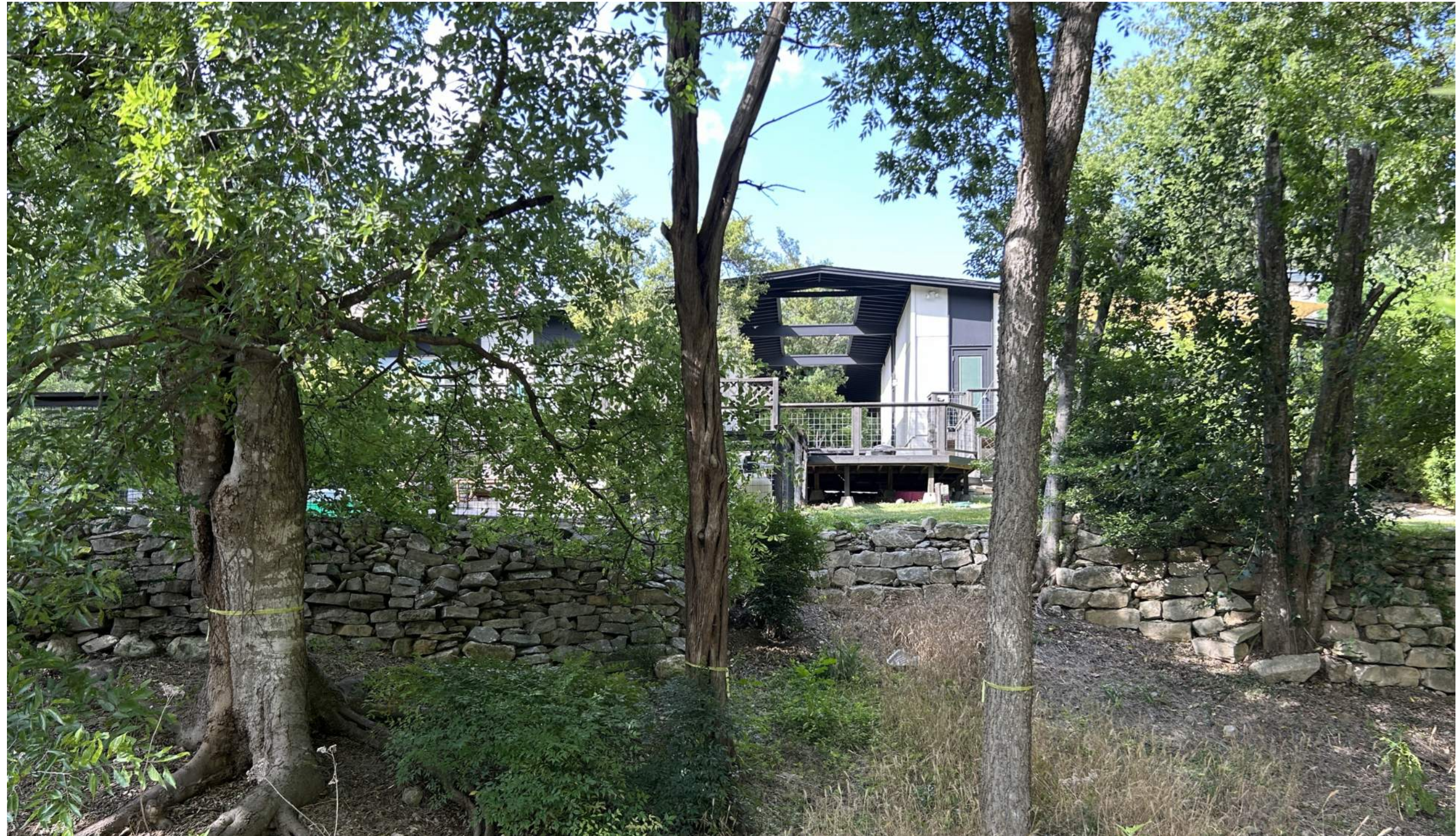
Existing Building Exterior
