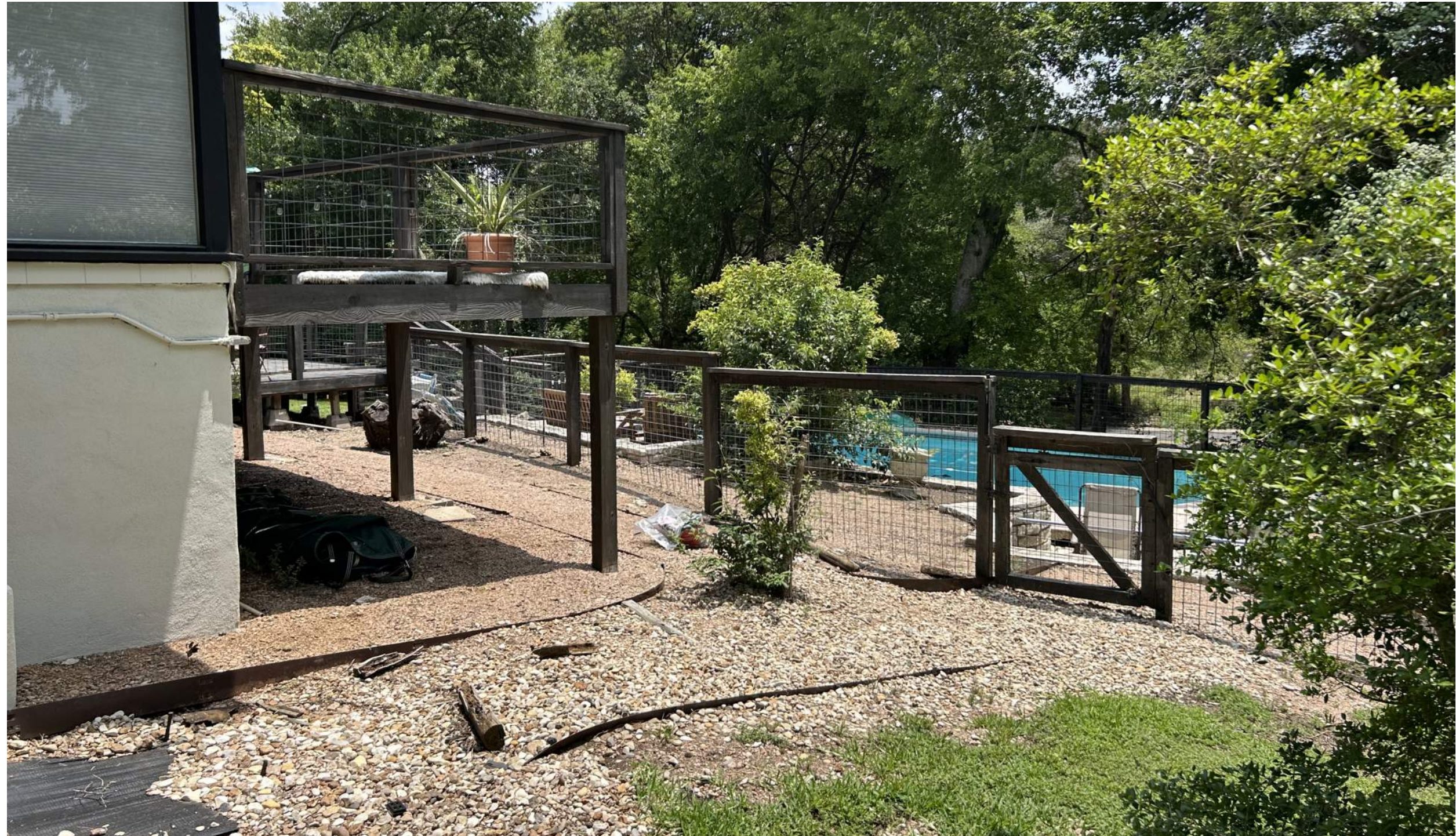
Existing Building Exterior
