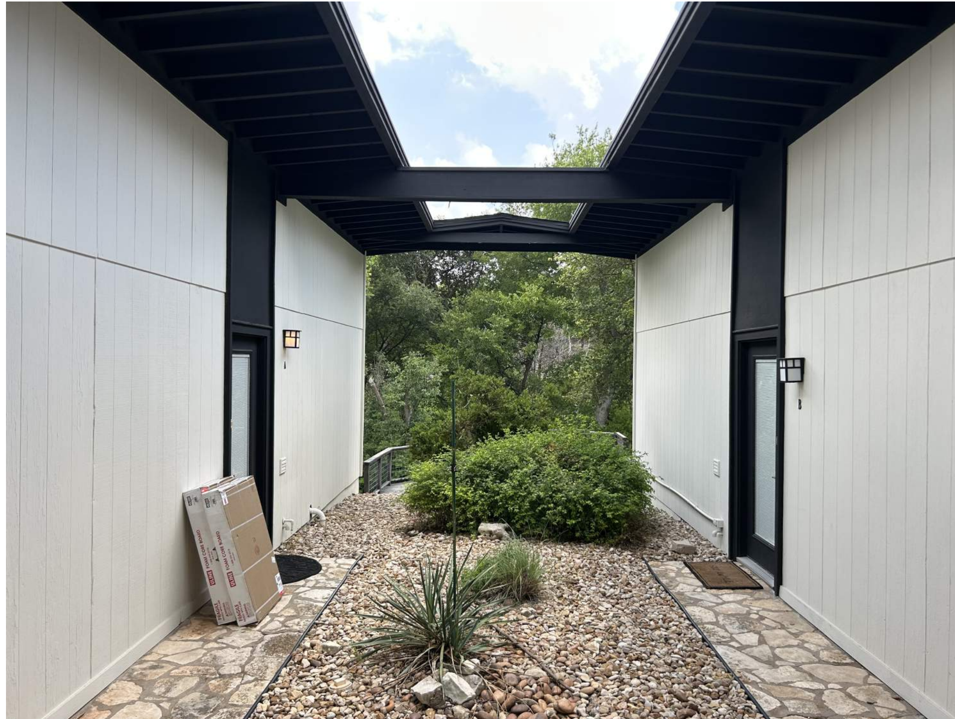
Existing Building Exterior
