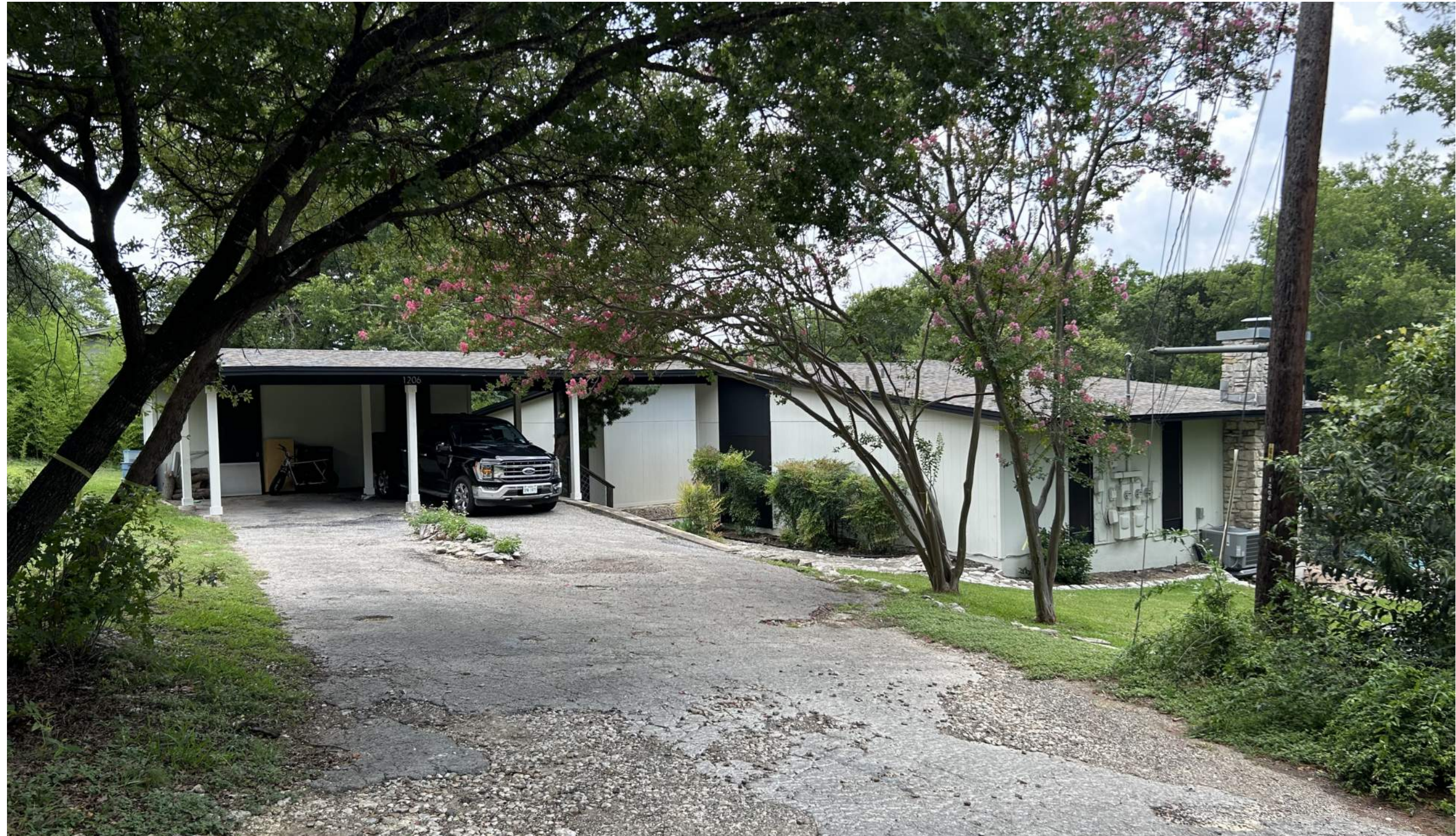
Existing Building Exterior
