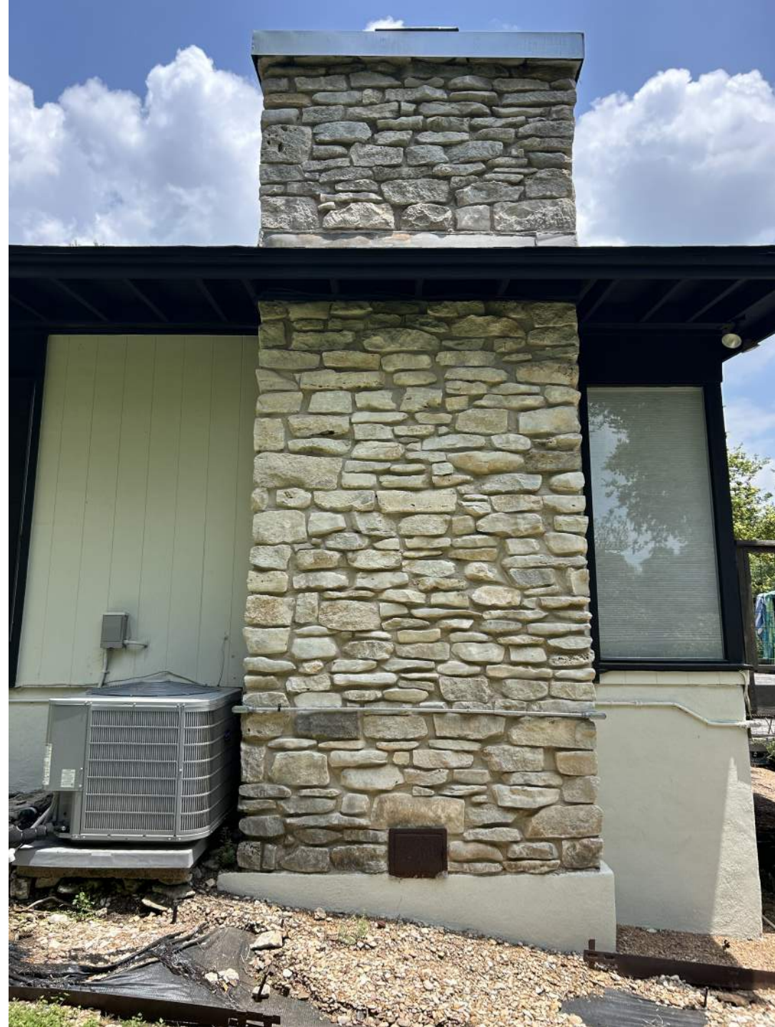
Existing Building Exterior
