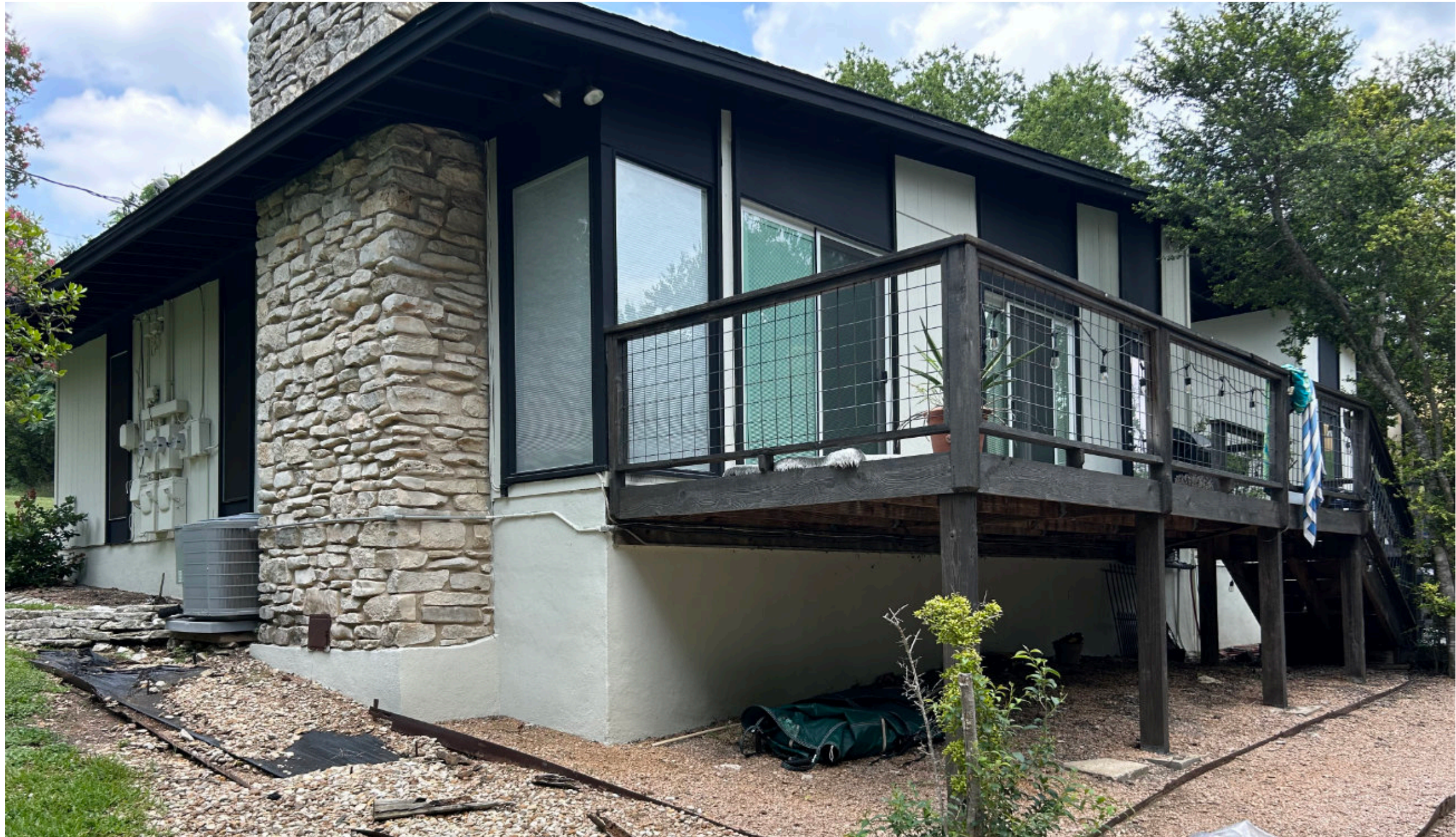
Existing Building Exterior
