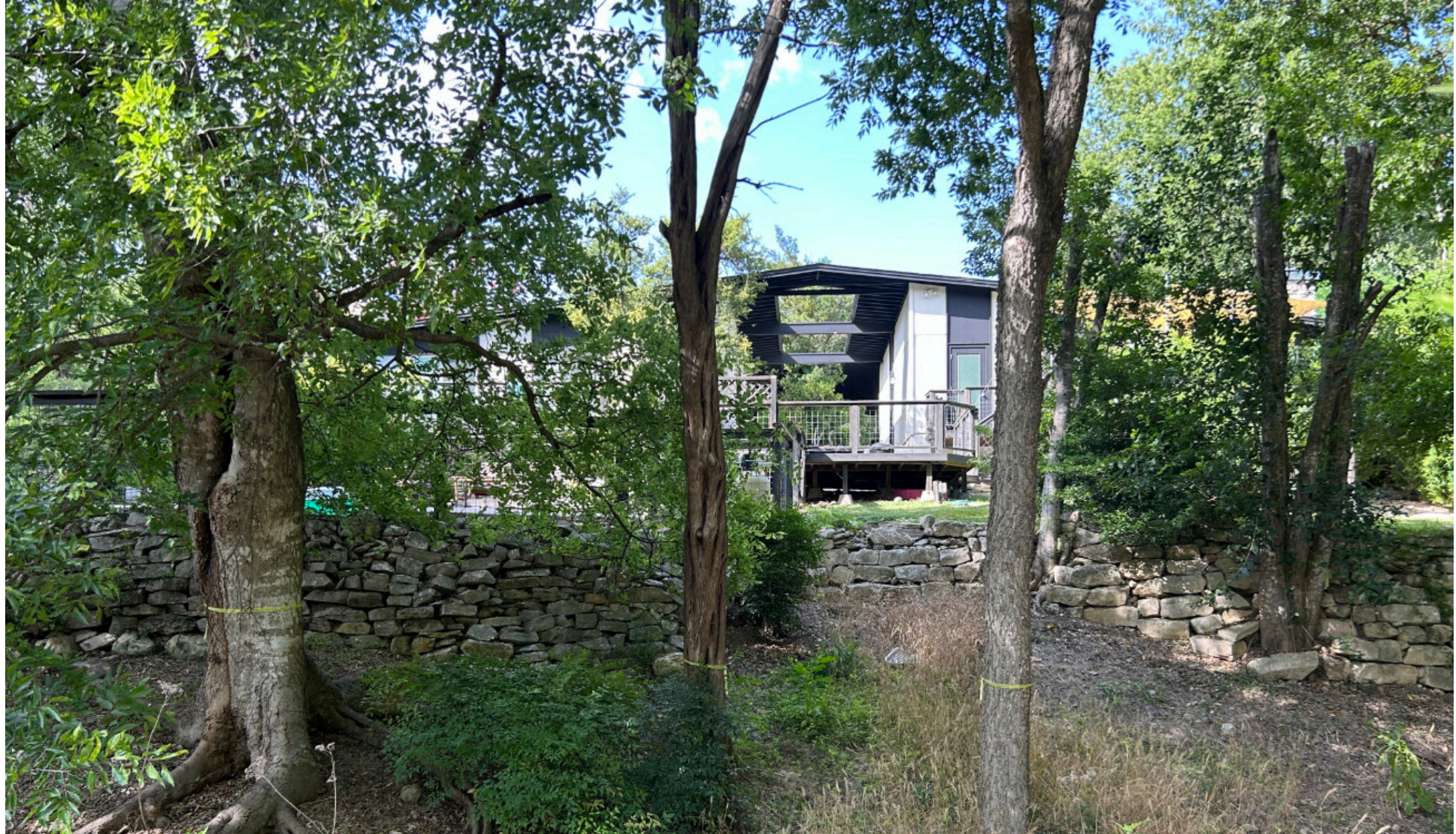
Existing Building Exterior
