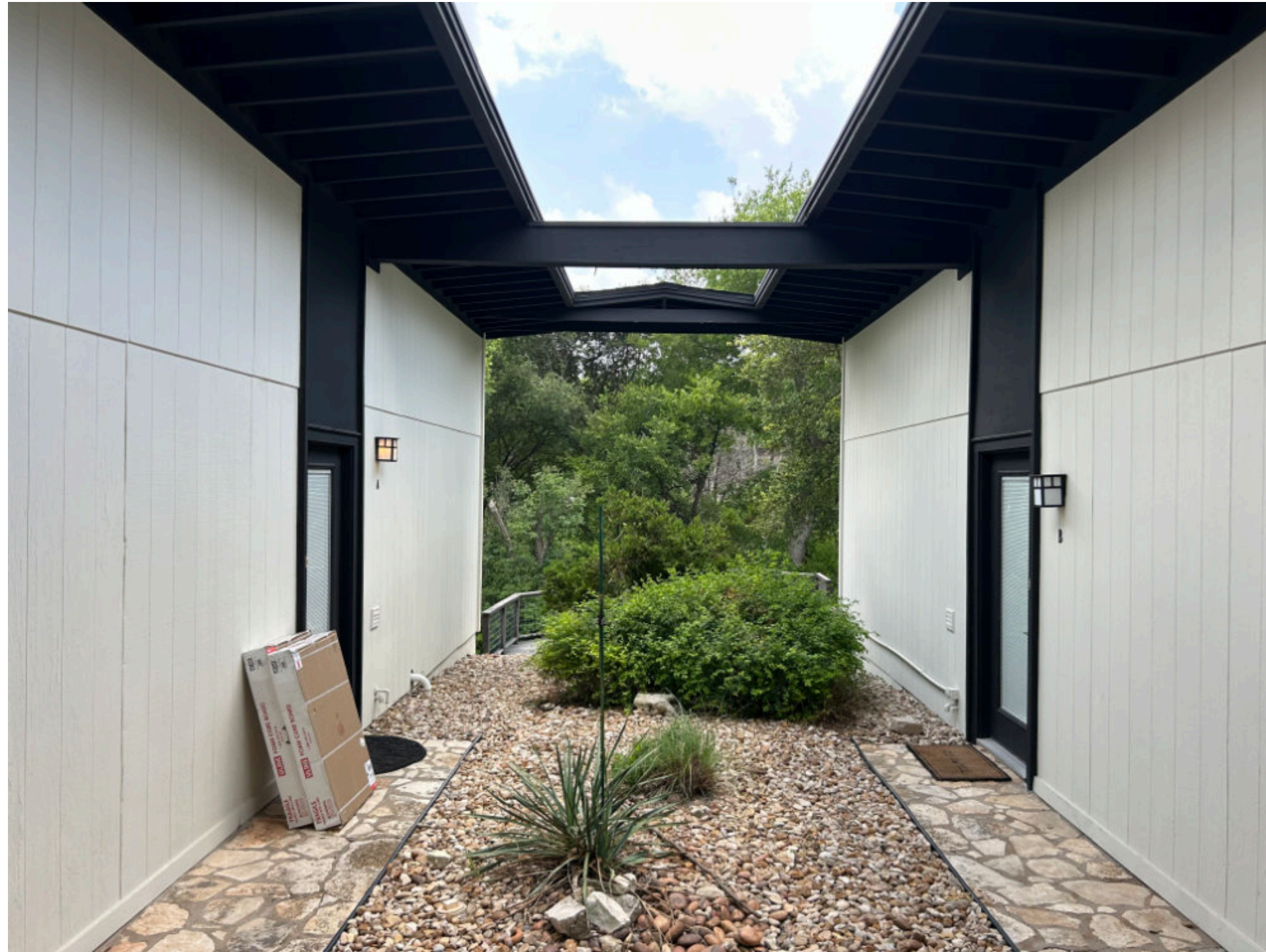
Existing Building Exterior
