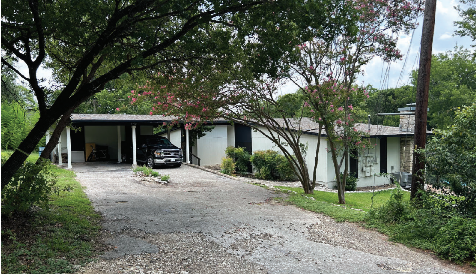
Existing Building Exterior
