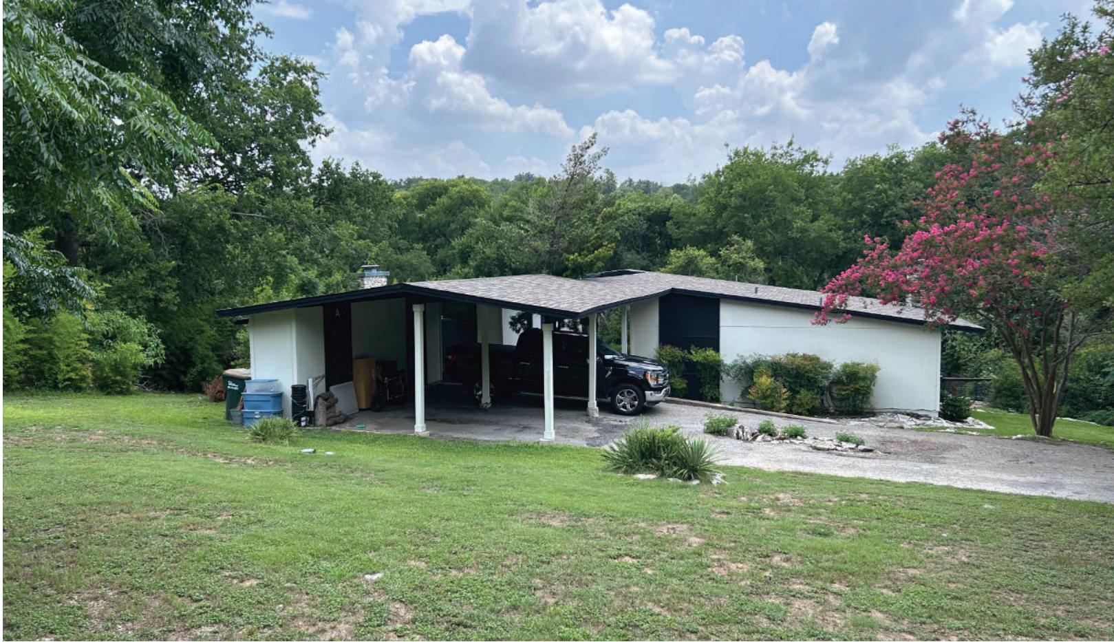
Existing Building Exterior
