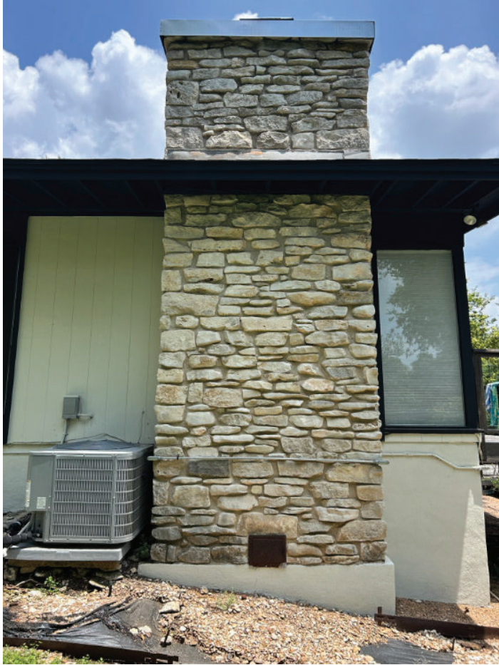
Existing Building Exterior
