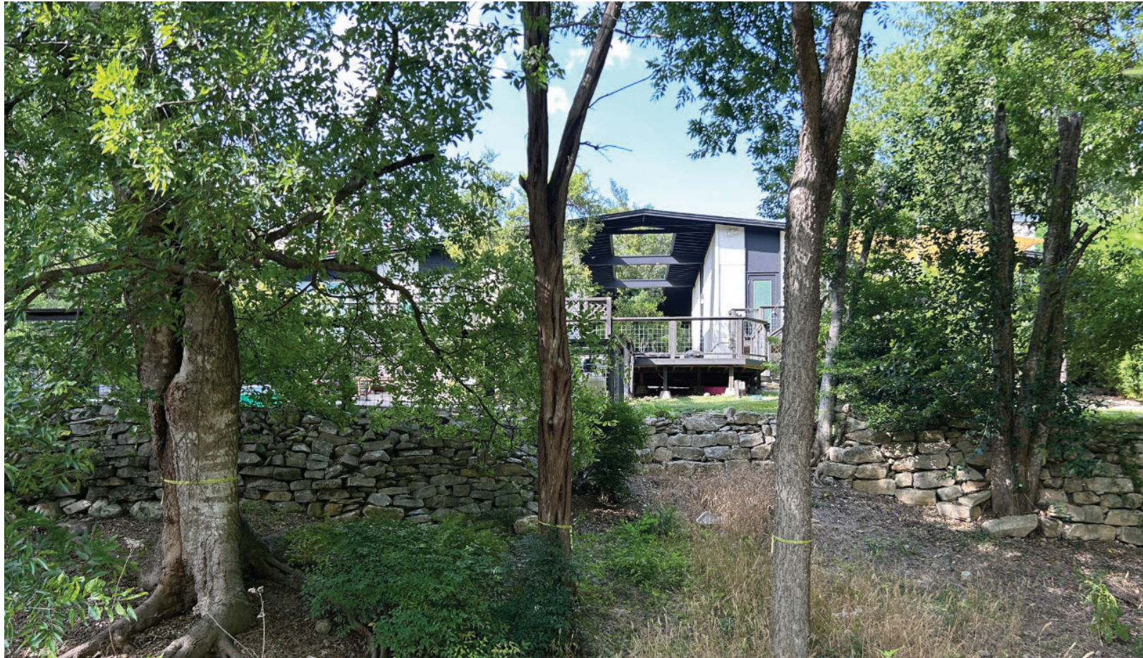
Existing Building Exterior
