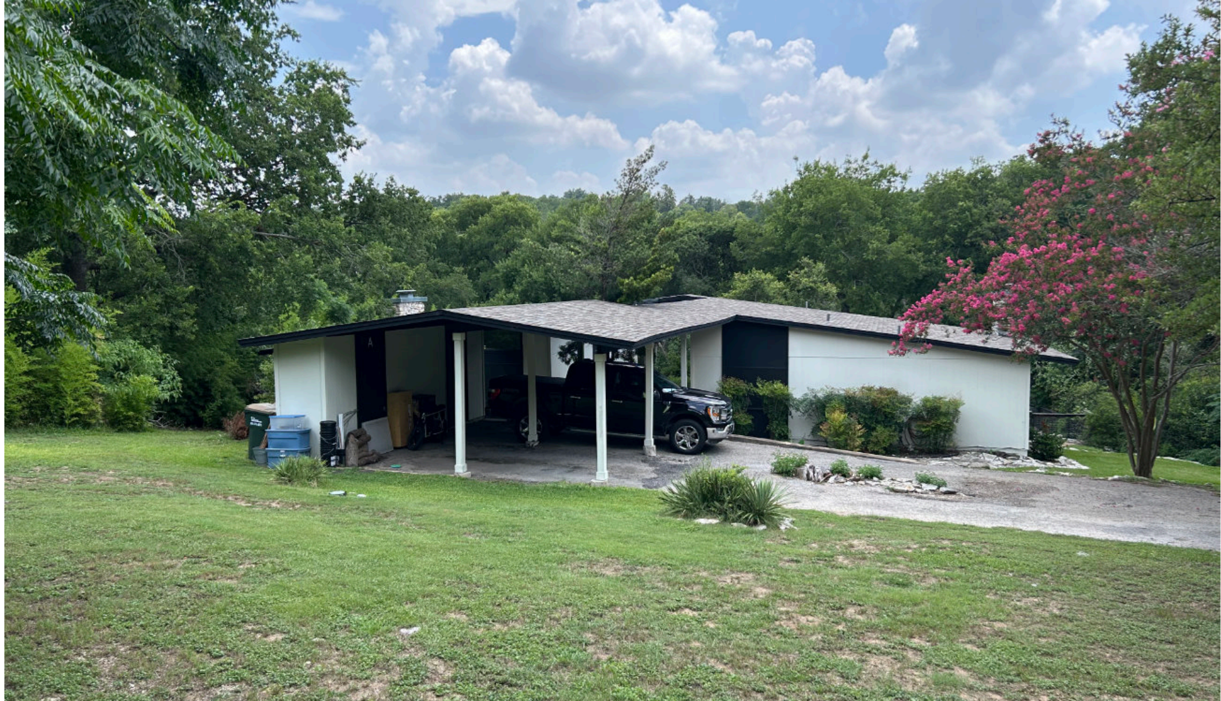
Existing Building Exterior
