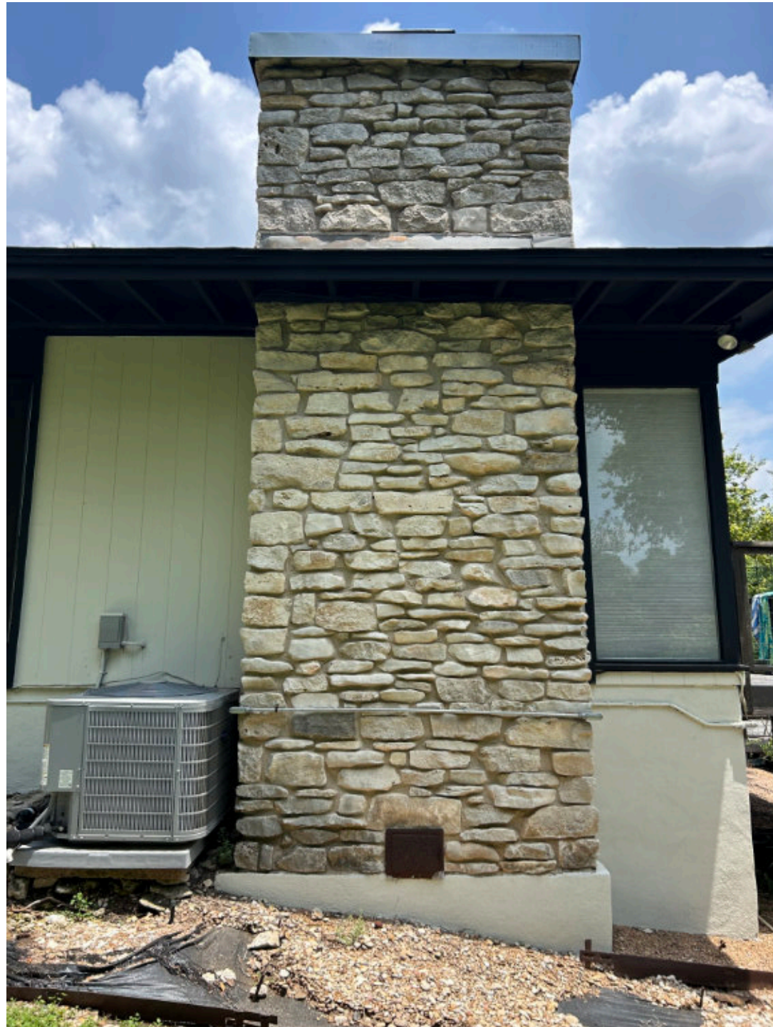
Existing Building Exterior
