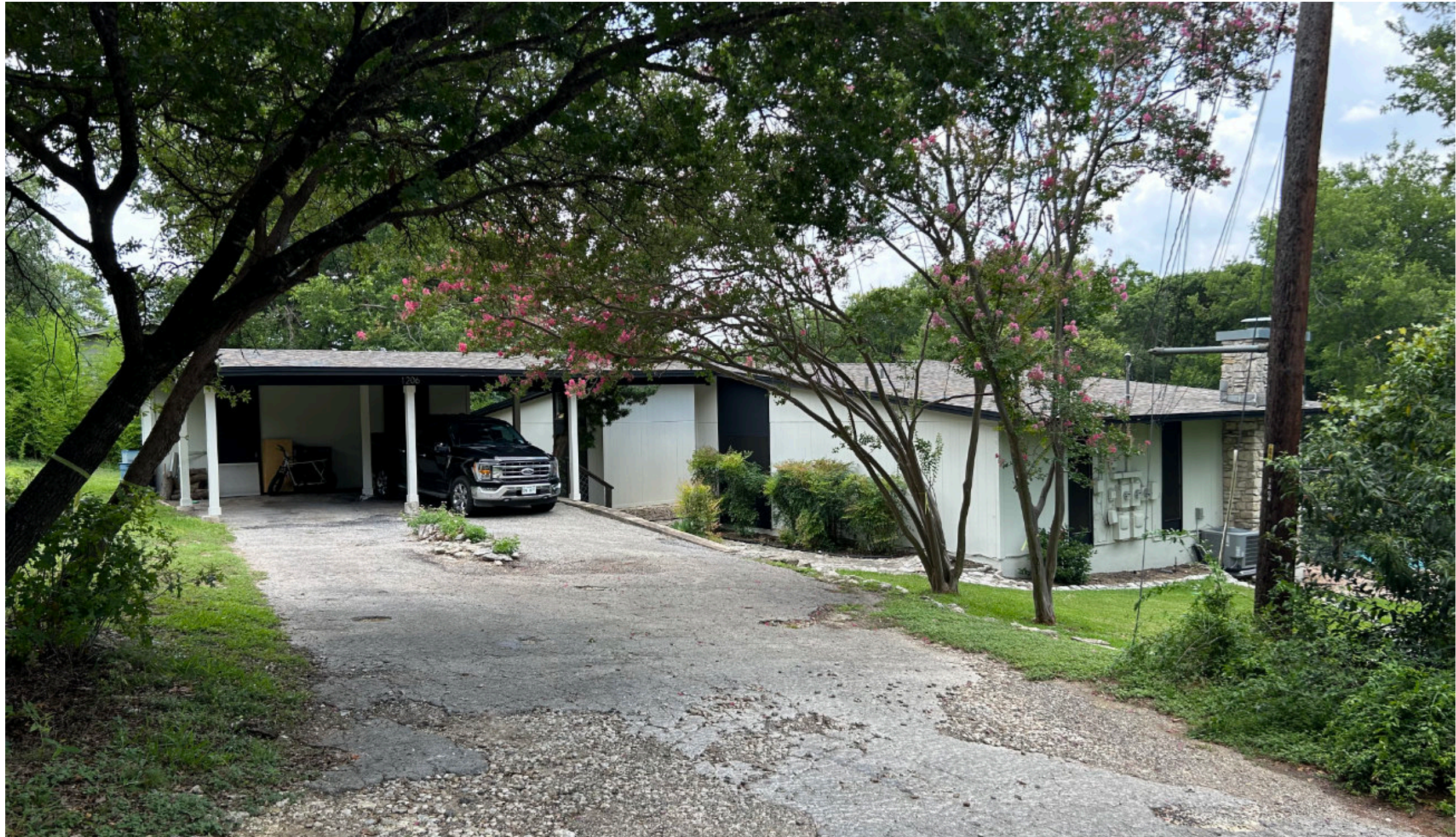
Existing Building Exterior
