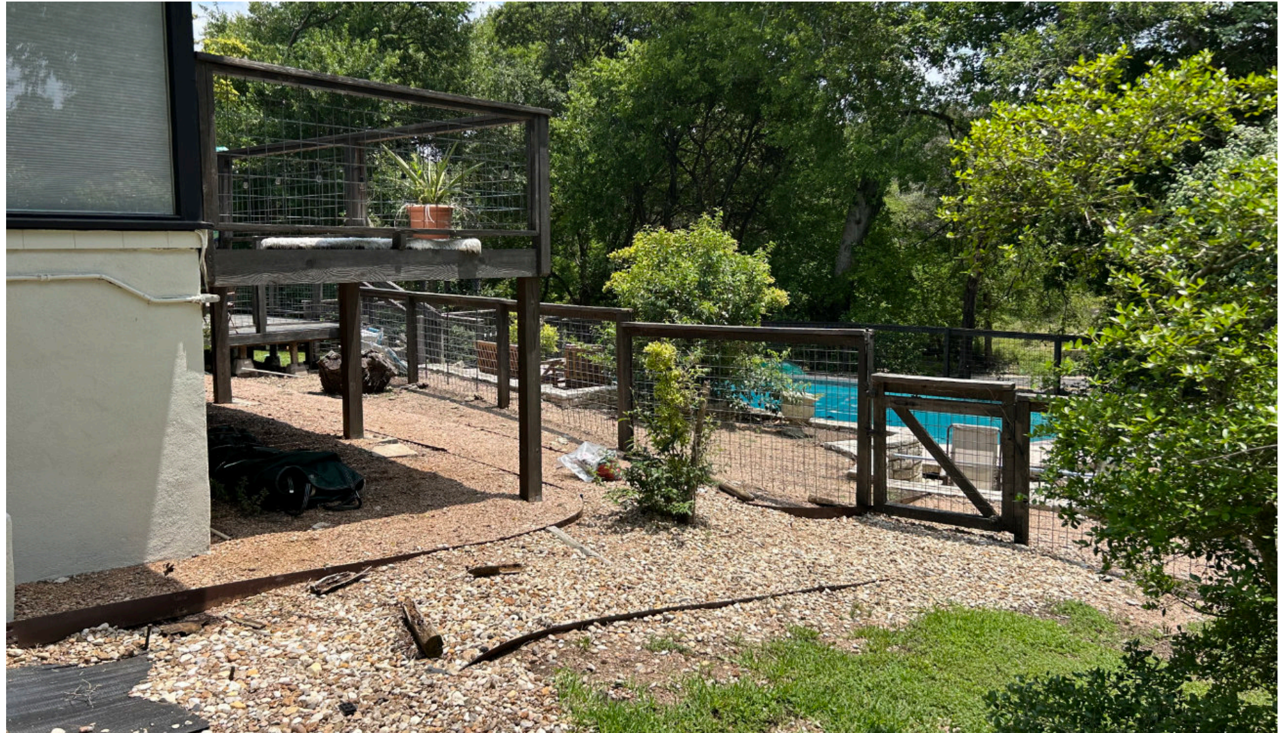
Existing Building Exterior
