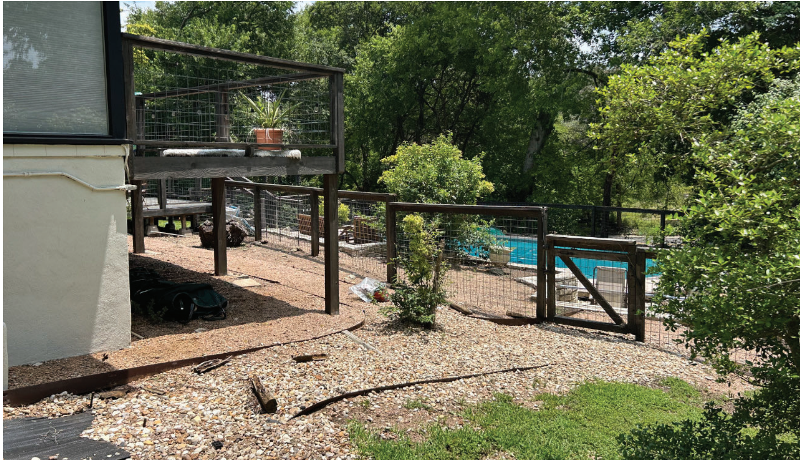
Existing Building Exterior
