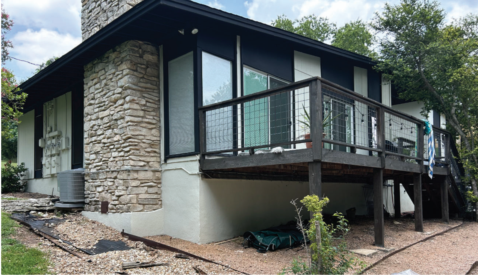
Existing Building Exterior
