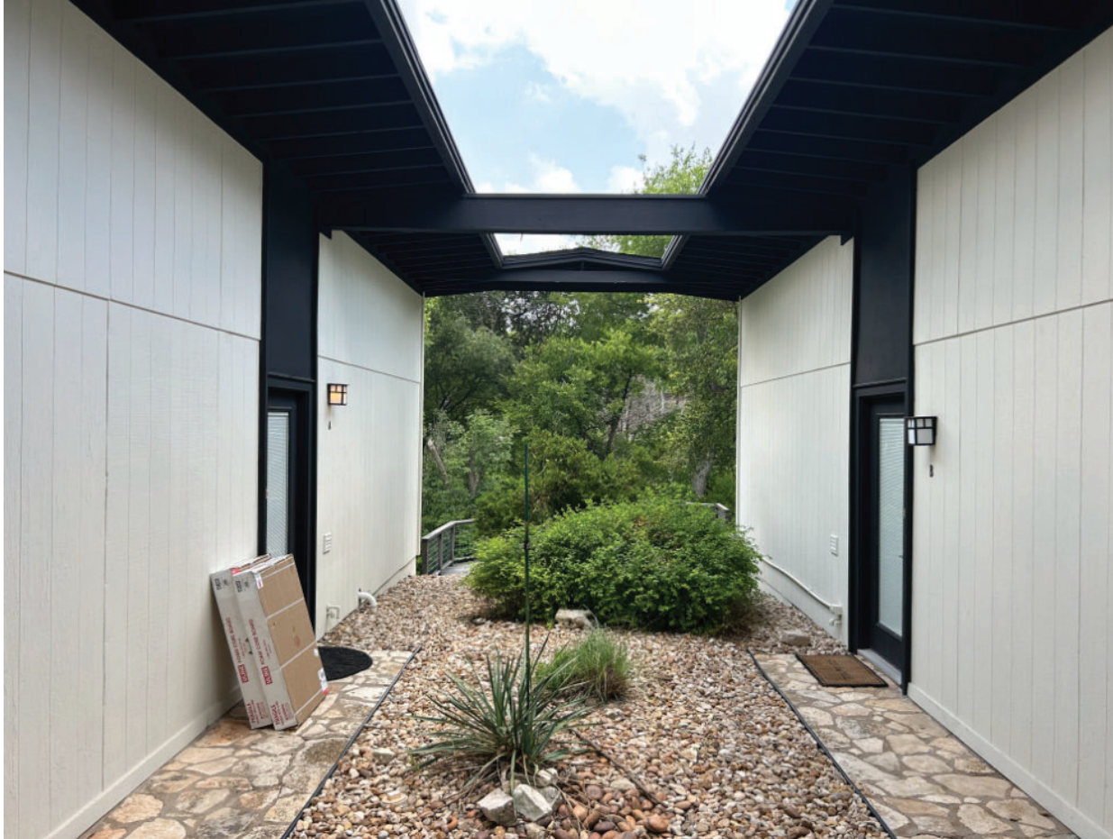
Existing Building Exterior
