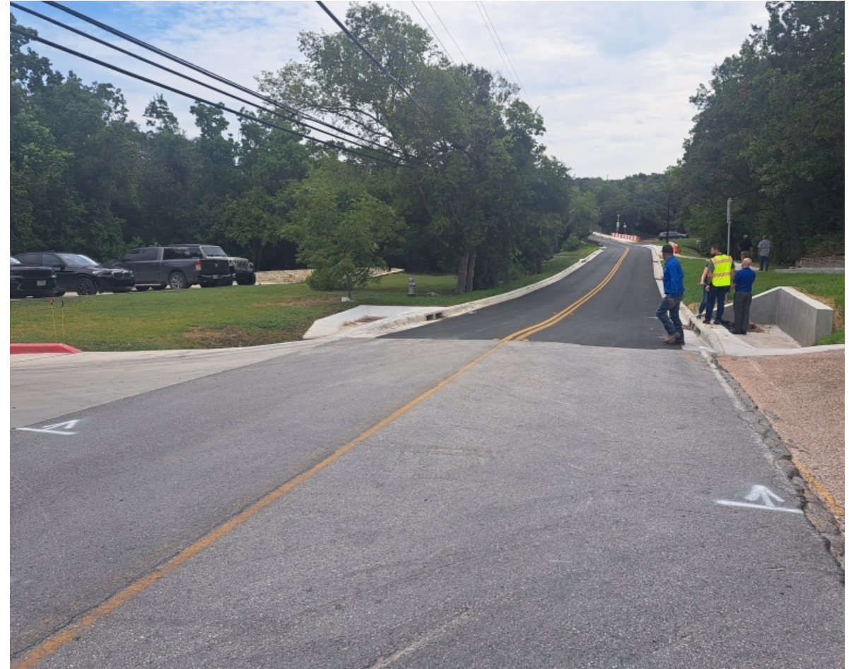
South connection to existing roadway
