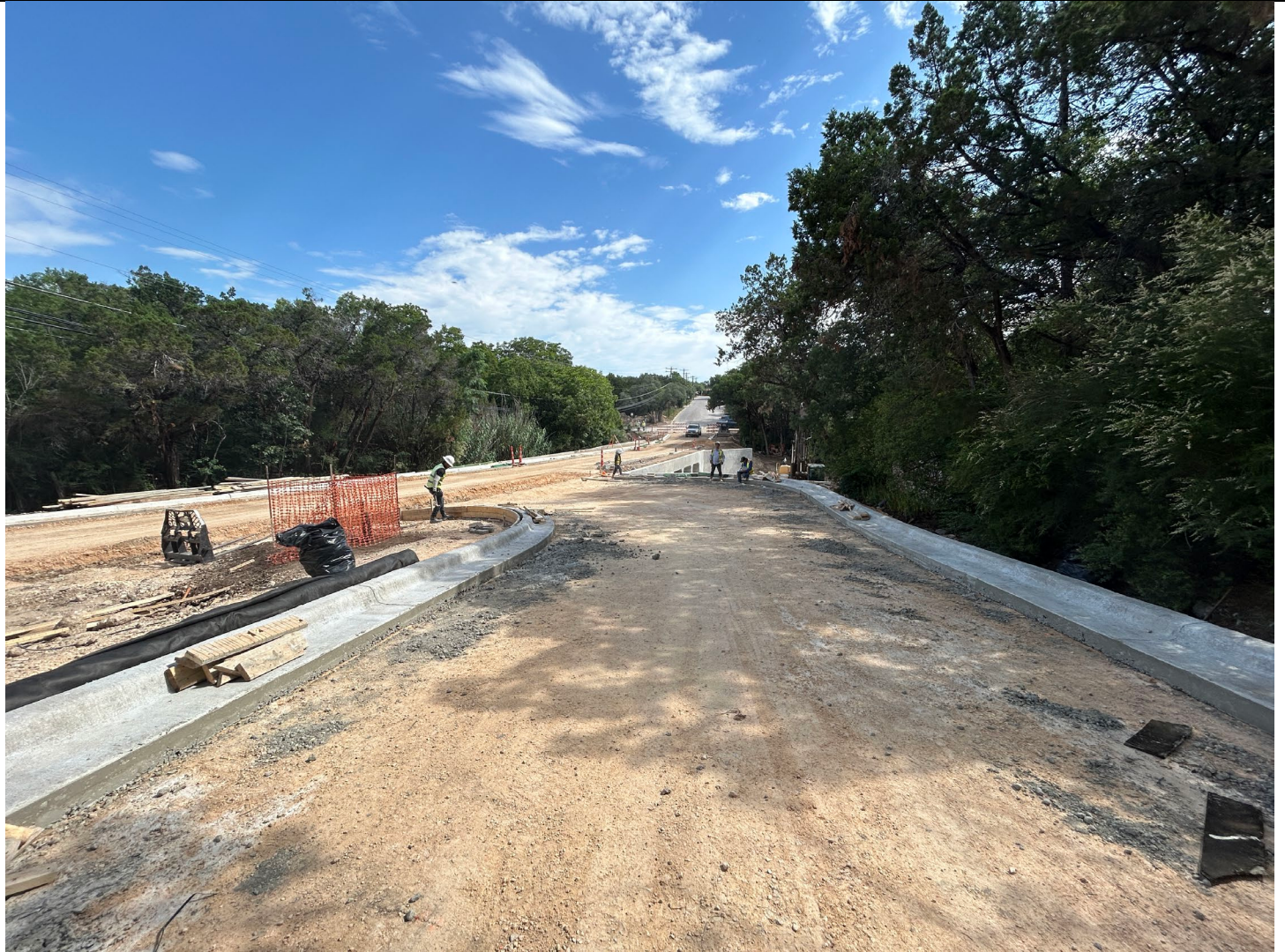
Figure 3: Phase 1 Segment (north end) looking north from private driveway
