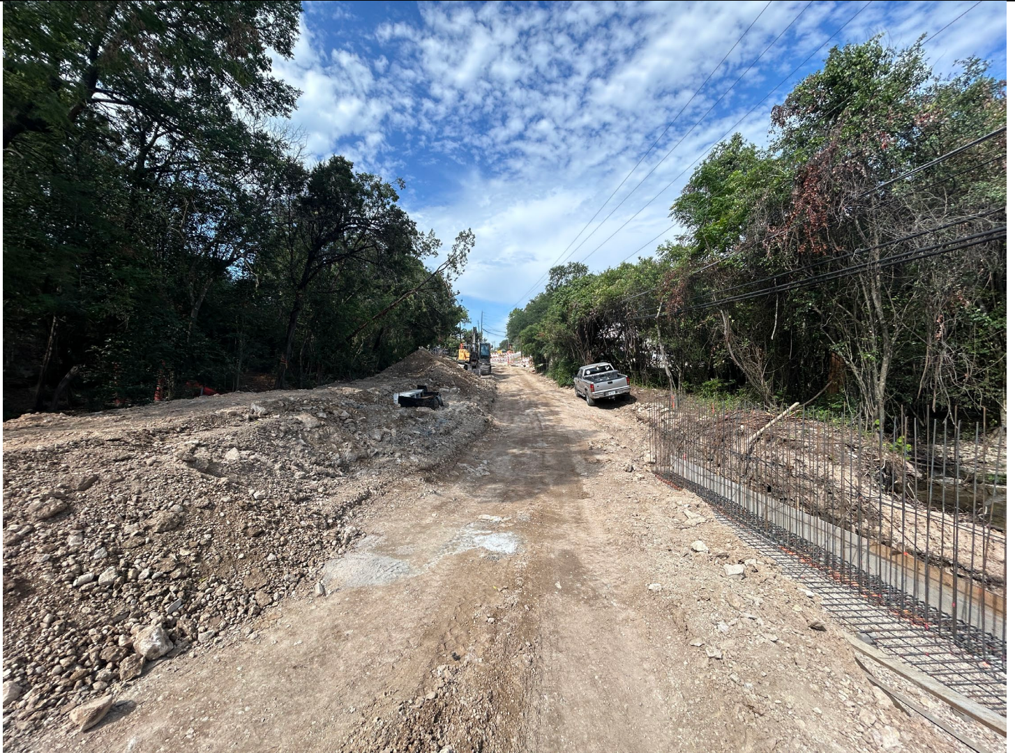
Figure 5: Phase II Segment (south end) looking south
