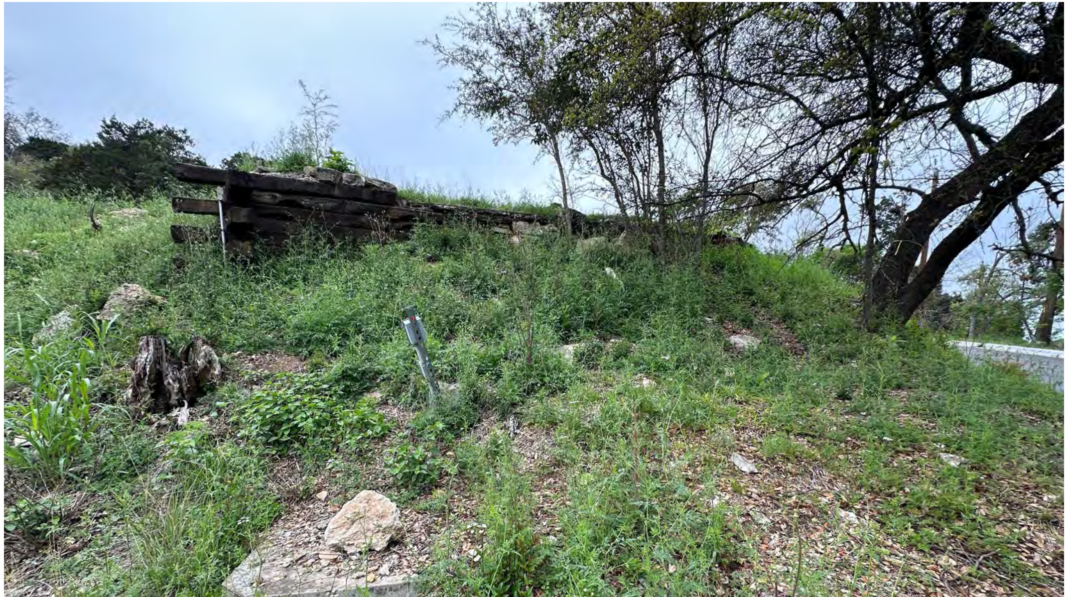
Existing timber retaining wall
