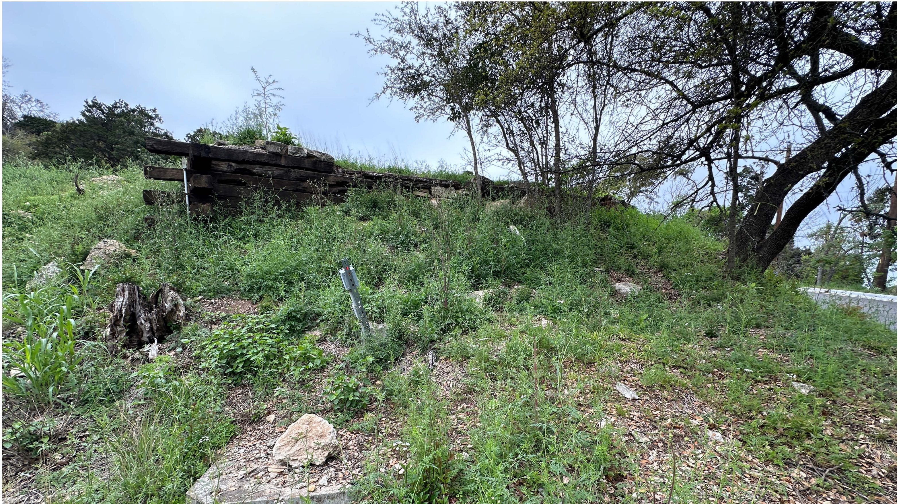
Existing timber retaining wall
