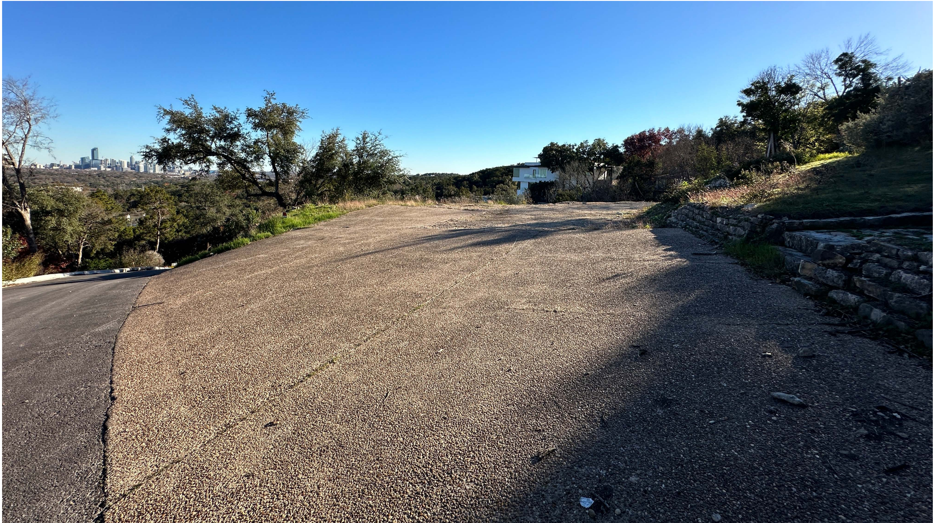
Previous house demolished / Existing drive & retaining walls (view from Harbor View)
