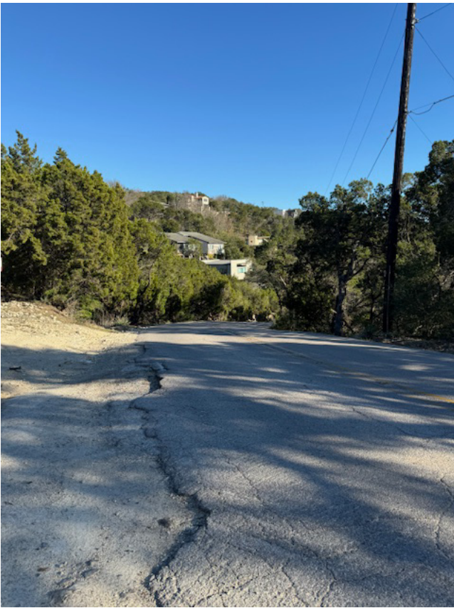
VIEW OF CONNECTION AT SKYLINE AND REDBUD
