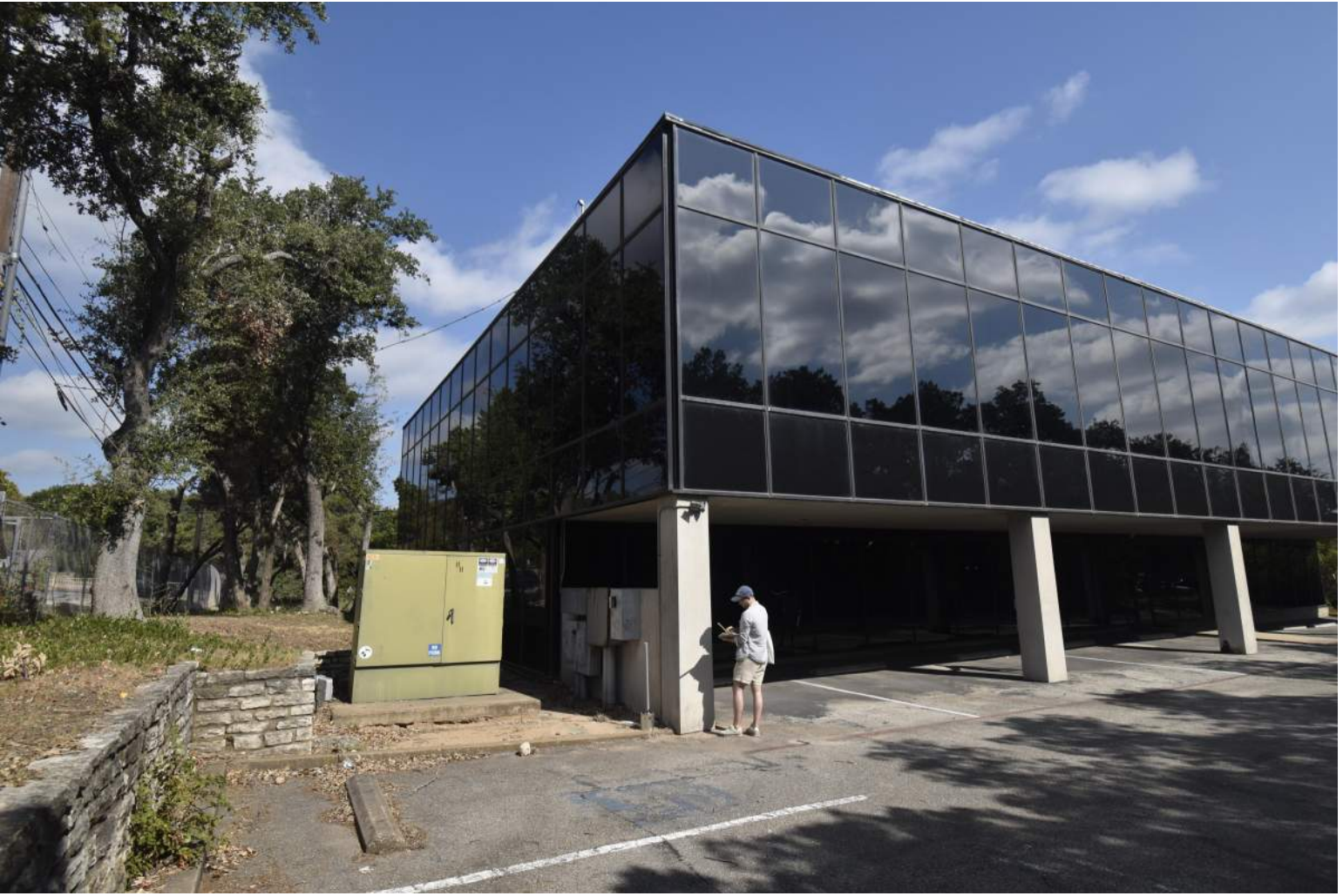
SE FACADE FACING
