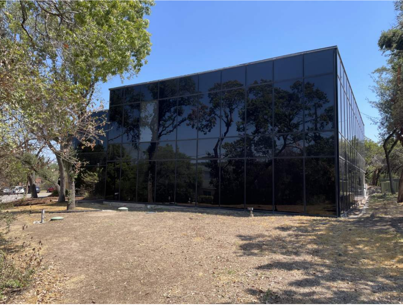
SW FACADE FACING WHS
