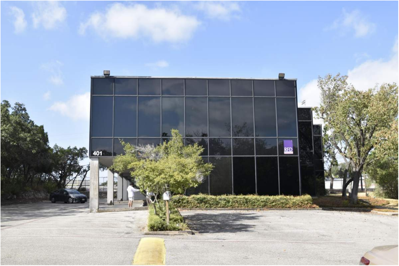
NE FACADE FACING PARKING
