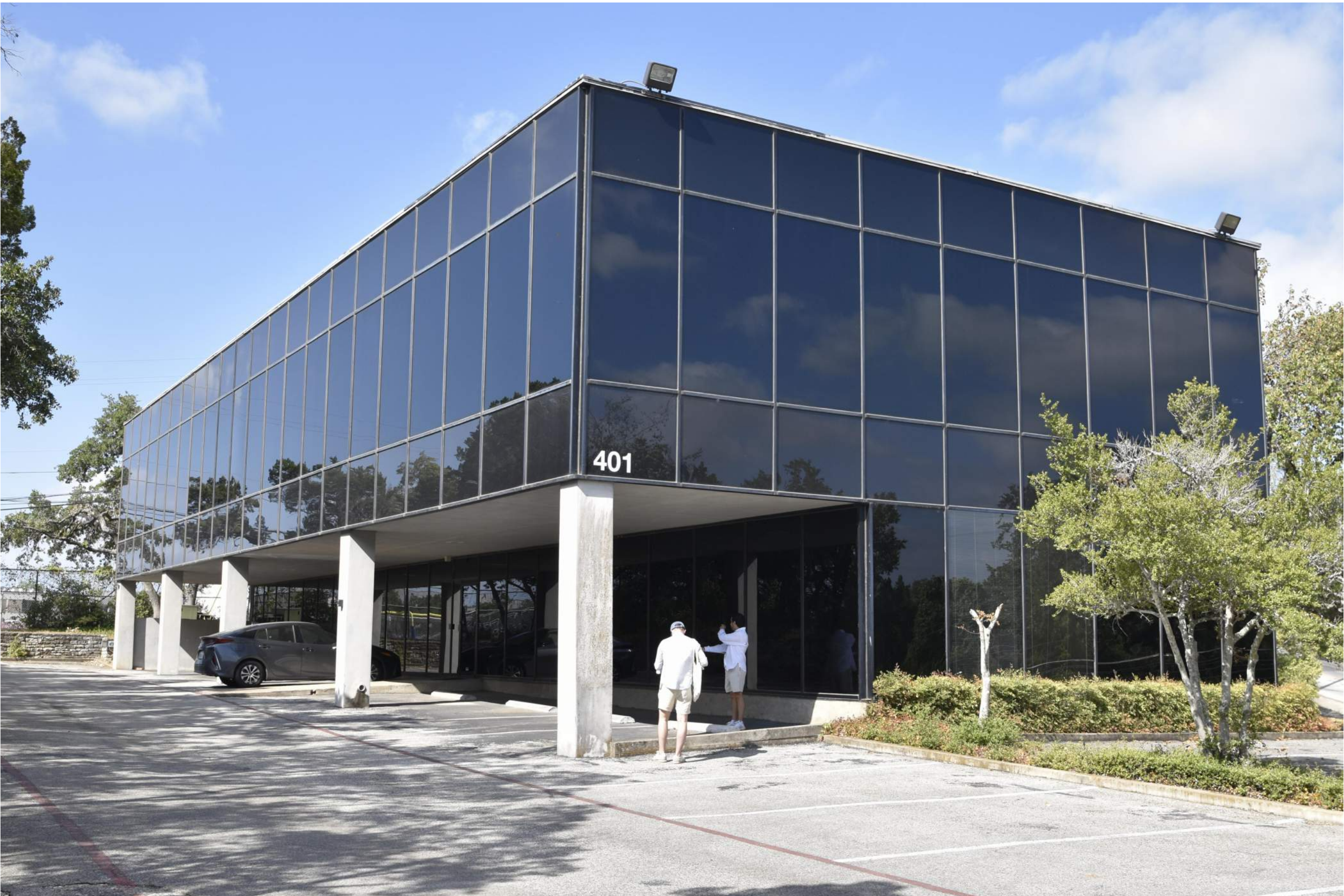
EXISTING REAR FACADE AND PARKING
