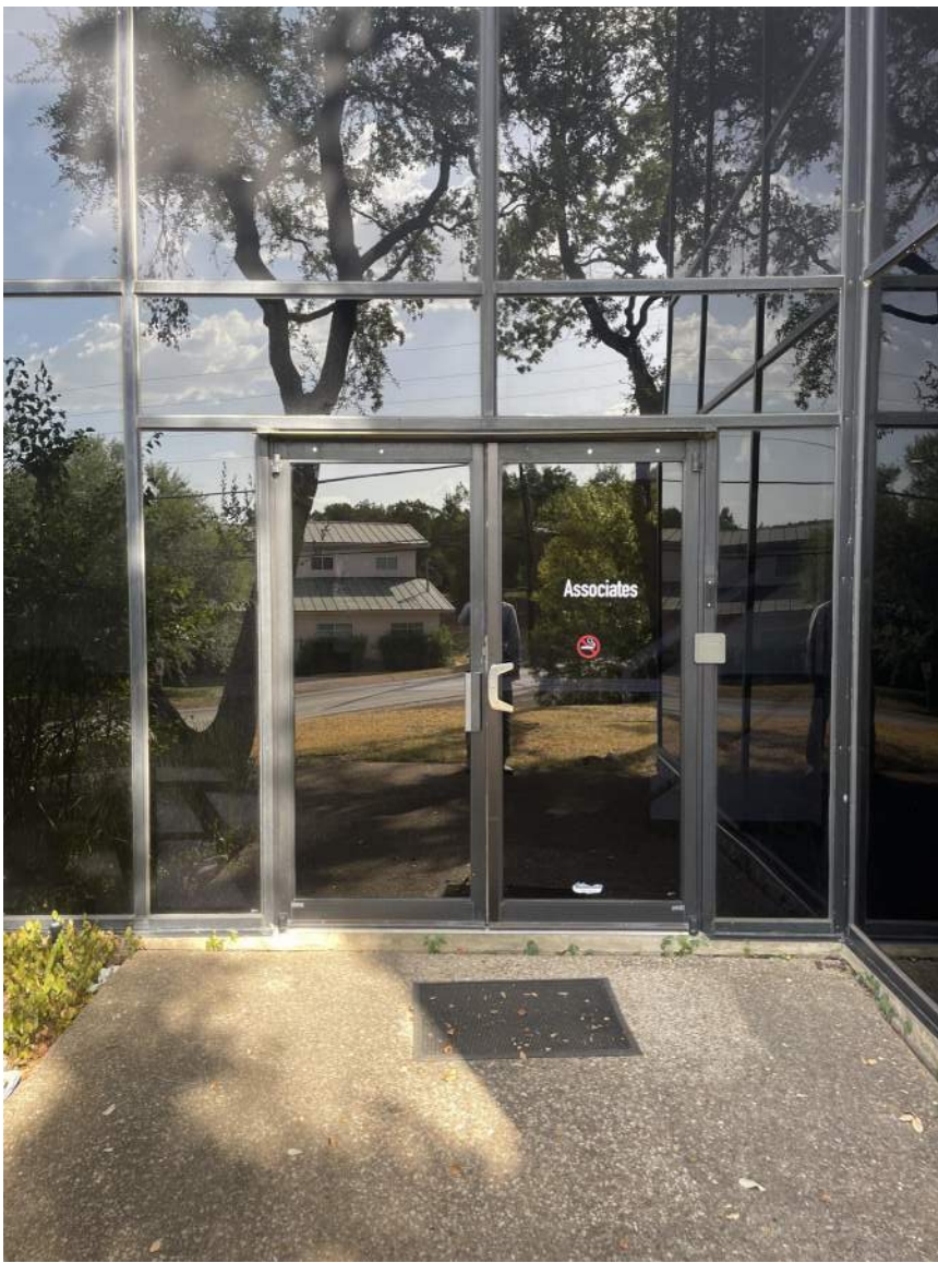
EXISTING ENTRY DOORS
