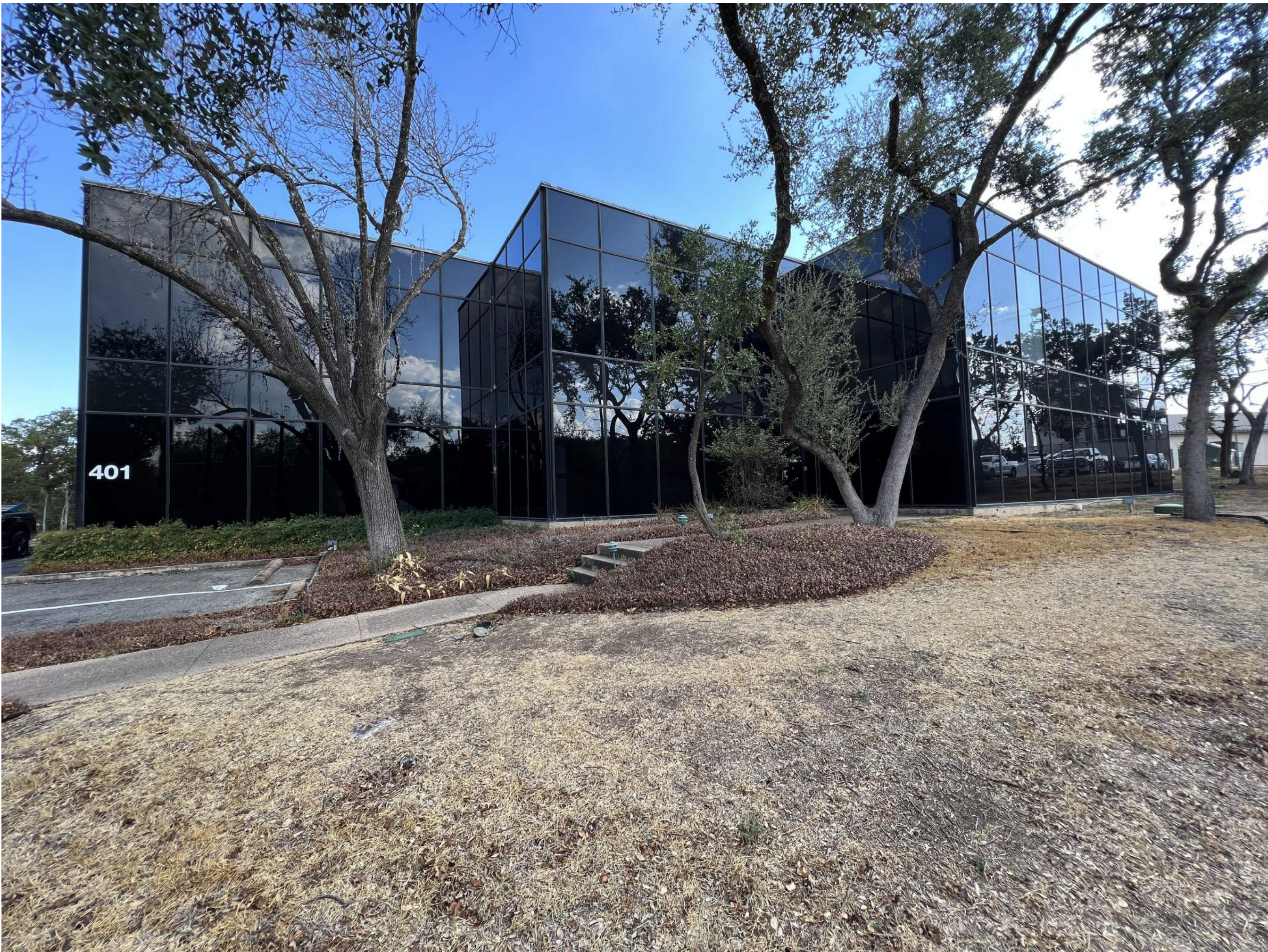
EXISTING FRONT FACADE
