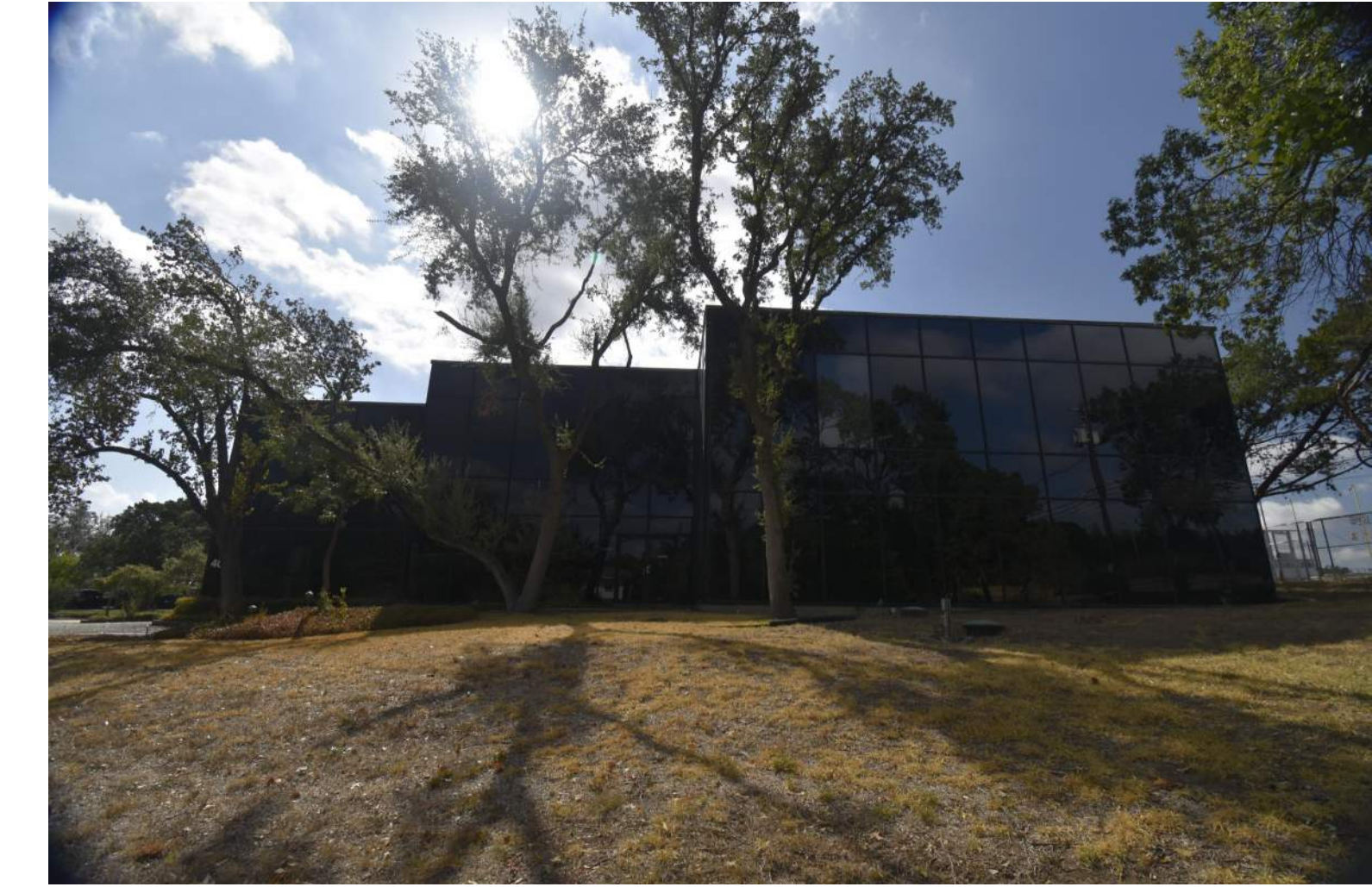
FACADE FACING CAMP CRAFT
