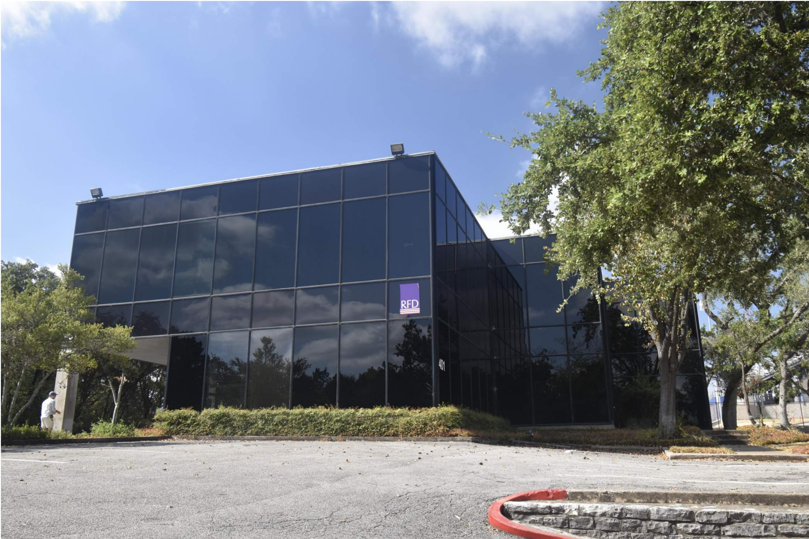
EXISTING NORTH EAST FACADE
