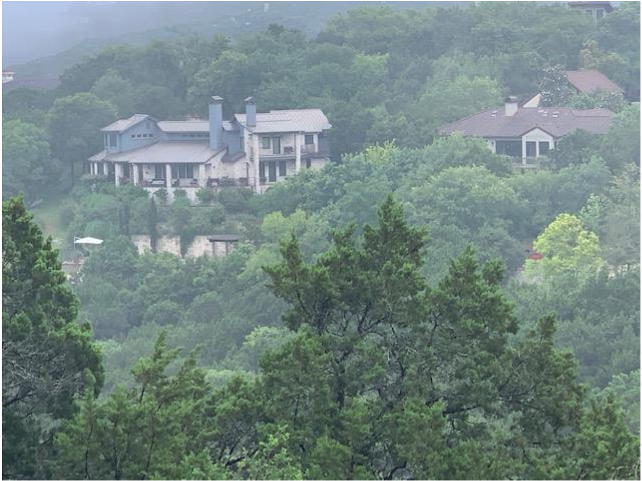
PICTURE 8: EXAMPLE OF NEIGHBORS ON OTHER SIDE OF VALLEY (ON WINDSONG) AND HOW THEY HAVE CONSTRUCTED SIMILAR RETAINING
