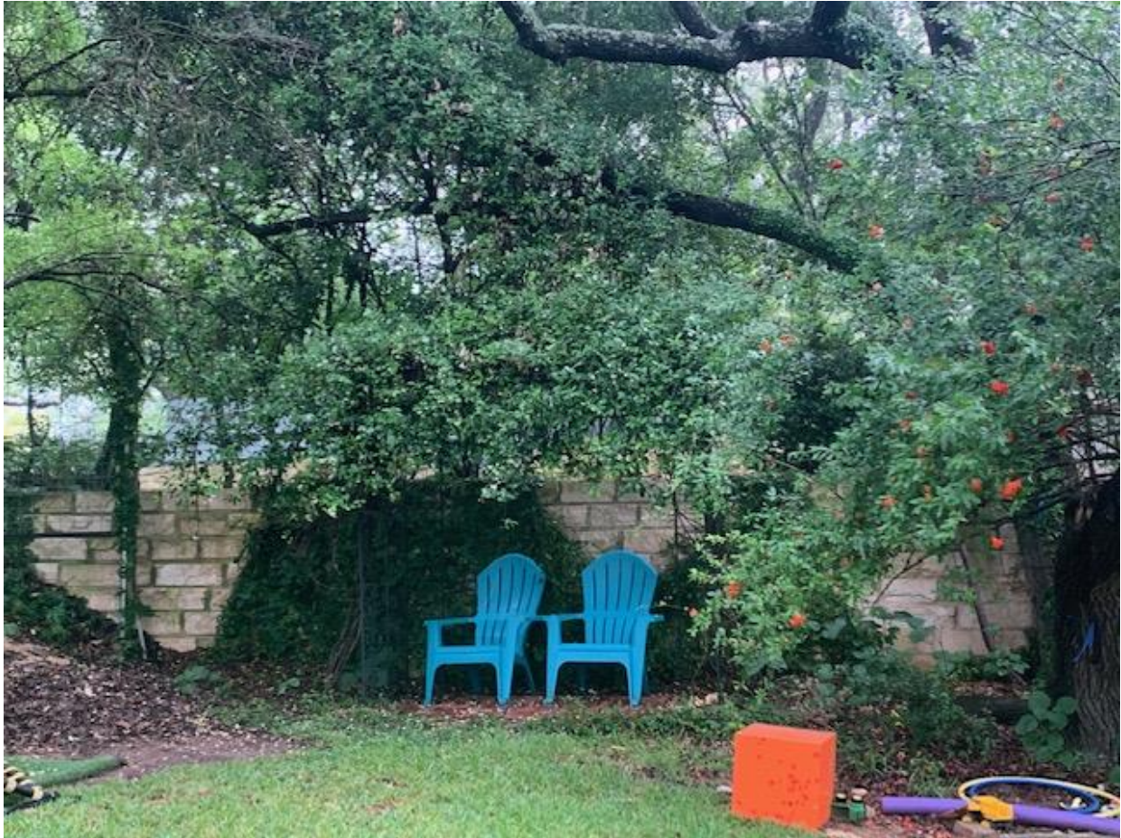
PICTURE 2: EXISTING RETAINING WALLS BETWEEN US AND NEIGHBORS AT 915 CALITHEA ROAD
