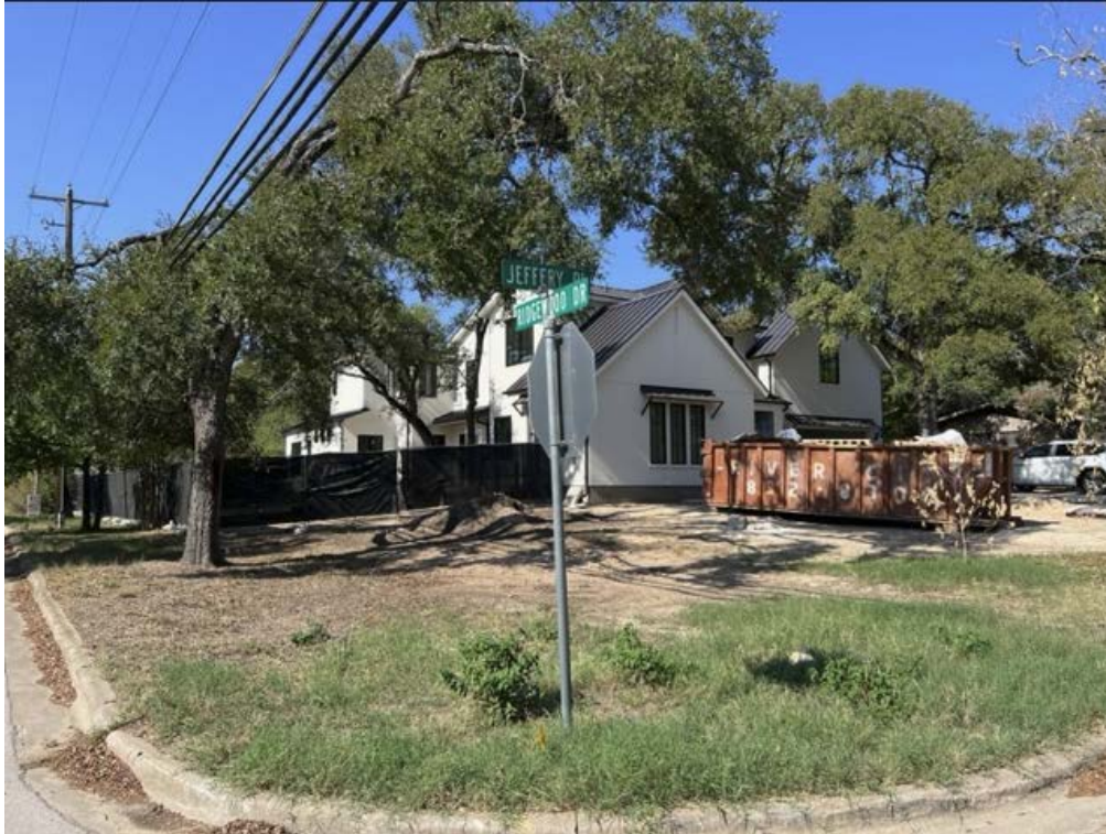
Existing construction fence placed at the property line at 5001 Jeffery Pl:
