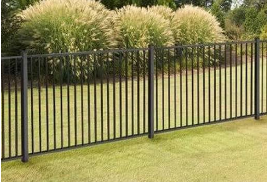
FENCE TYPE F2, 6' HT. AVERAGE BLACK PICKET FENCE TO MATCH EXISTING STYLE WITH FLAT TOP AND BOTTOM RAILS
