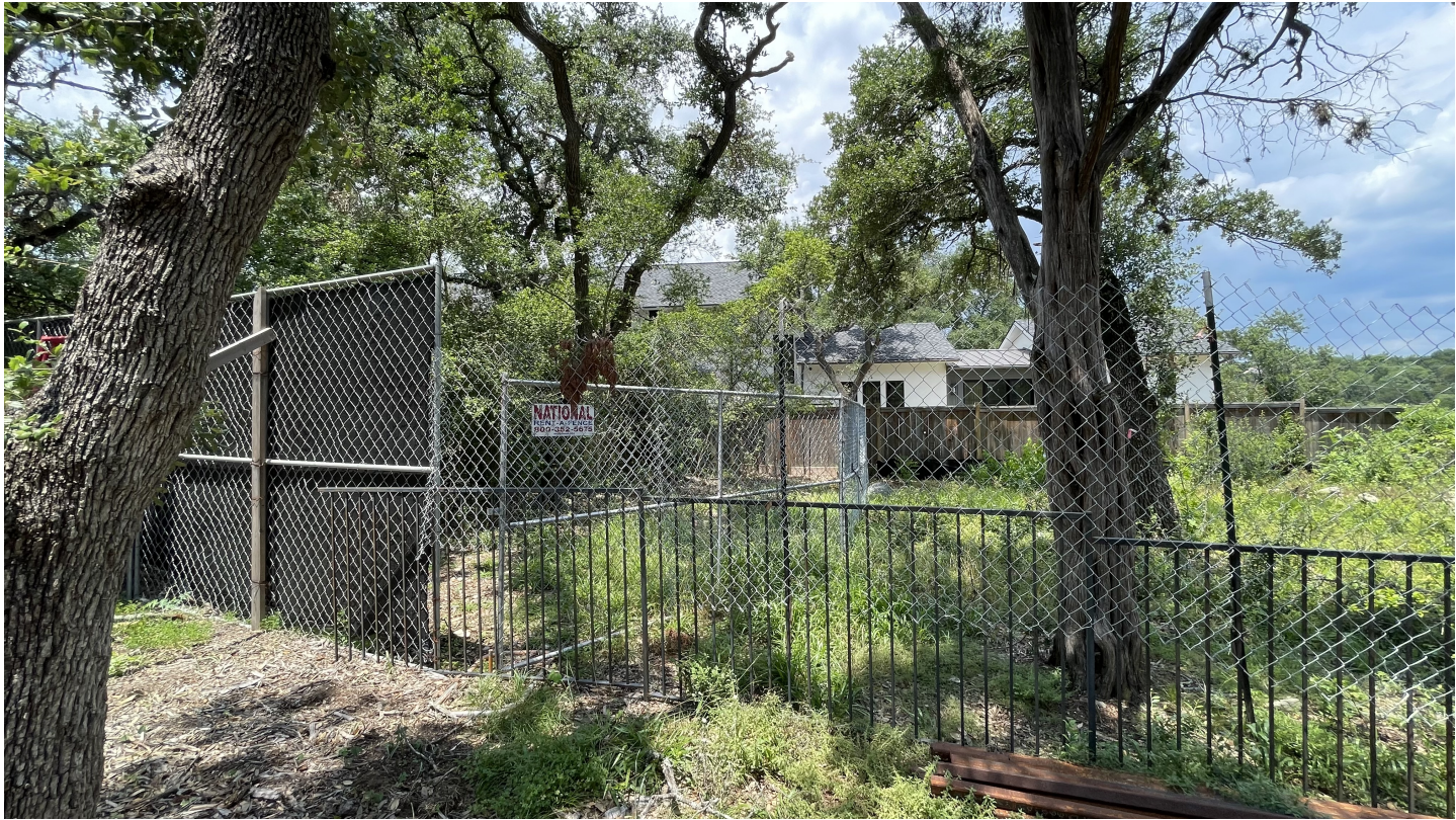
1. 902 / 904 LIVE OAK CIRCLE PROPERTY LINE FENCING
