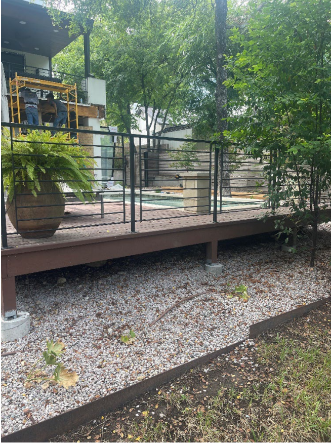
Figure 2- Existing Deck Elevation - Deck is 22 inches from grade on the point closest to the ground, 28 inches from grade on the tallest point.
